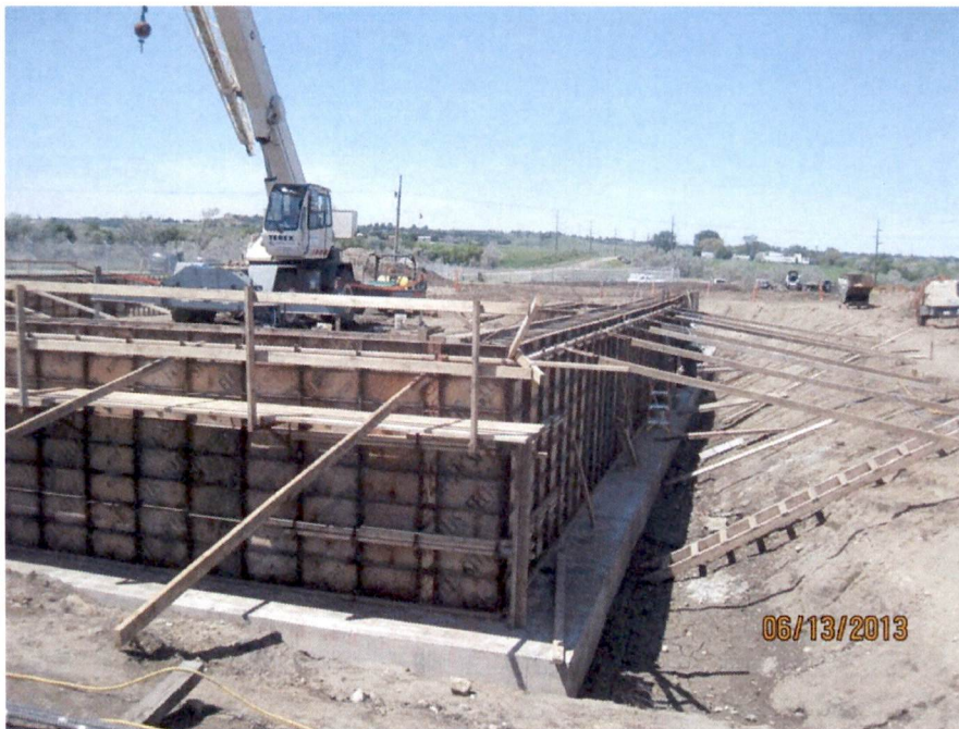
Service Building forms (looking SW)
