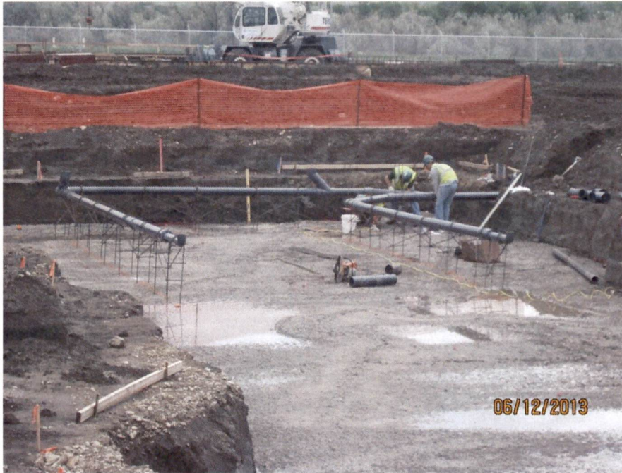
Drain Pipe installation in turbine foundation (looking S)
