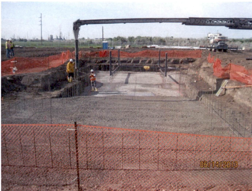
Turbine Foundation mud mat (looking S)
