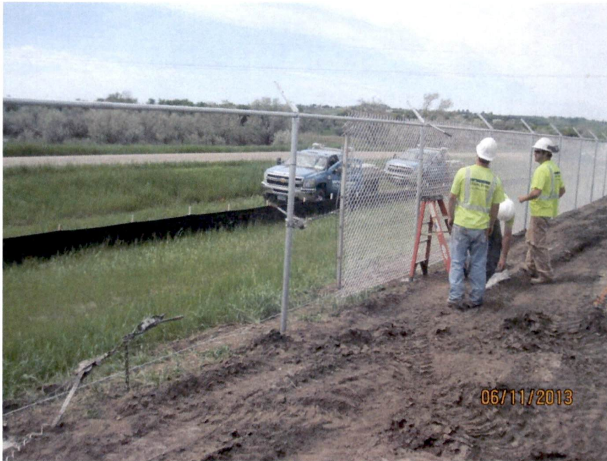
Site Security Fence installation (looking SW)
