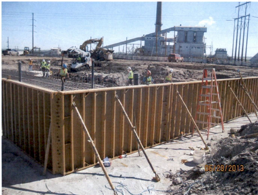
Combustion turbine forms and rebar (looking NE)
