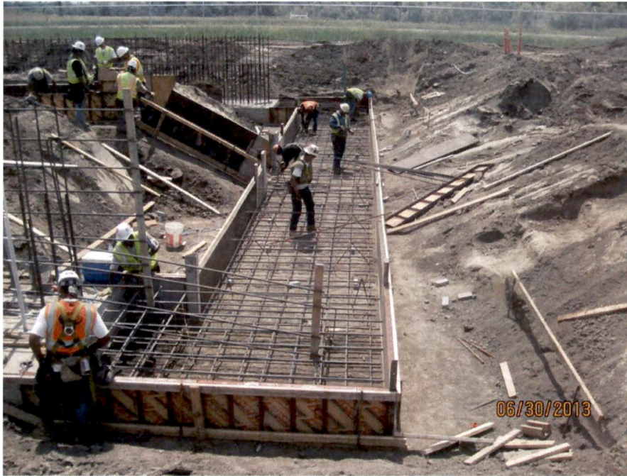
Service Building footer (looking S)
