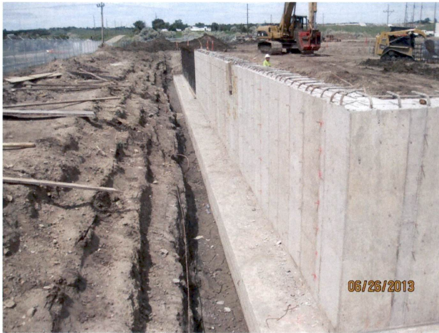
Service Building wall (looking W)
