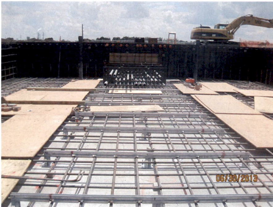
Electrical conduit embedments at Combustion turbine (looking S)
