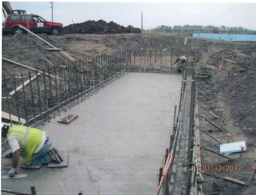
Foundation slab of PEECC (looking S)
