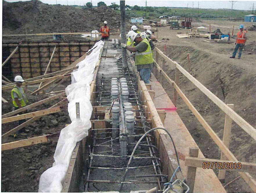
Service Building grade beam (looking W)
