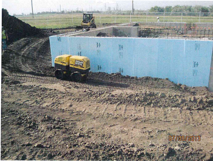
Backfill around Service Building wall (looking S)
