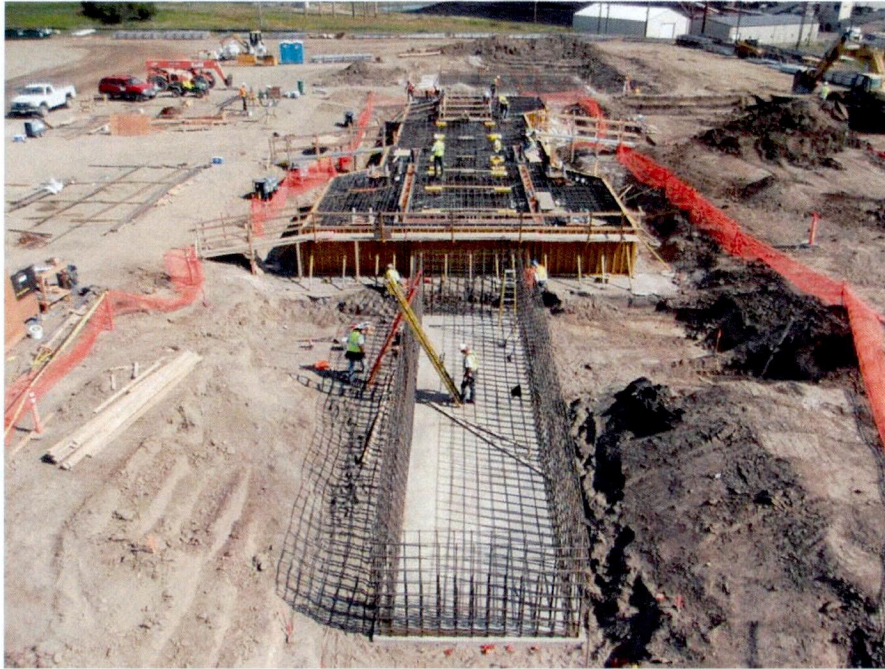
Combustion turbine and PEECC foundation (looking N)
