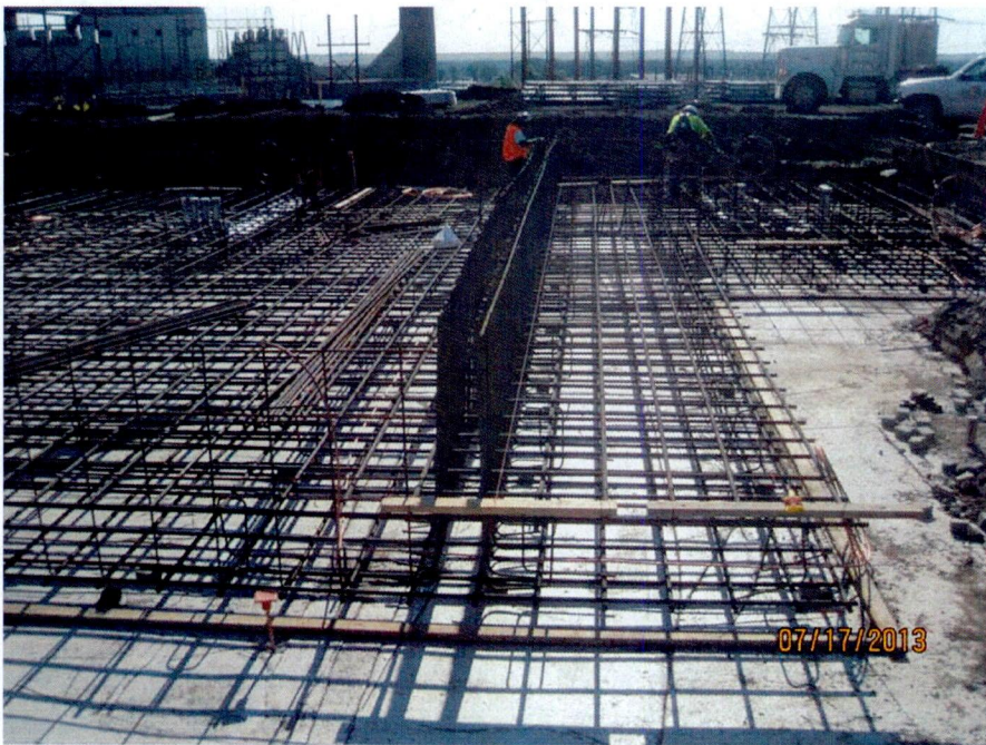
Rebar installation for GSU/UAT foundation (looking E)
