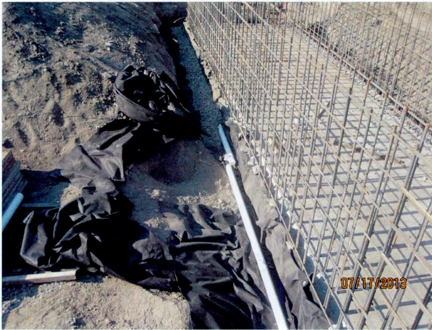
Perforated pipe installation for PEECC foundation (looking S)
