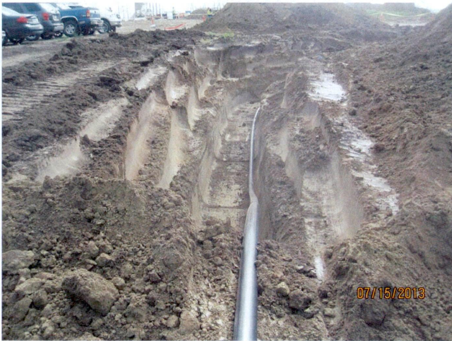
Potable water installation (looking E)
