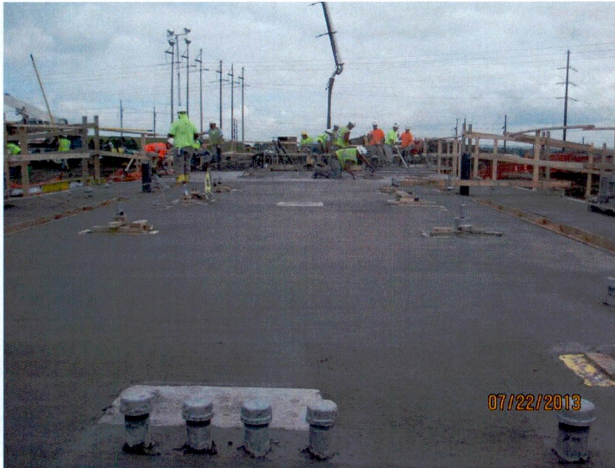
Combustion turbine foundation concrete placement (looking N)
