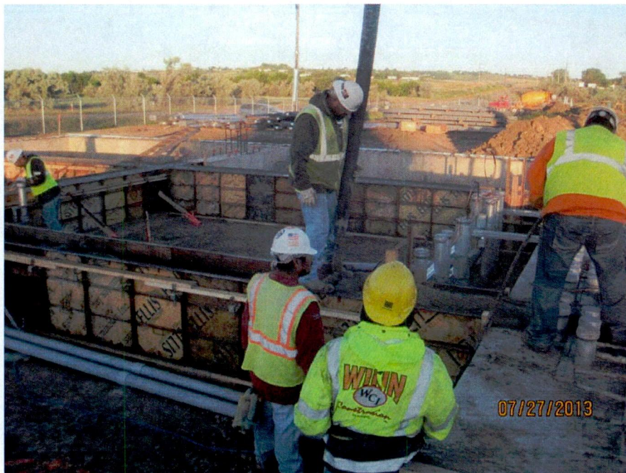
Service Building grade beam concrete placement (looking W)
