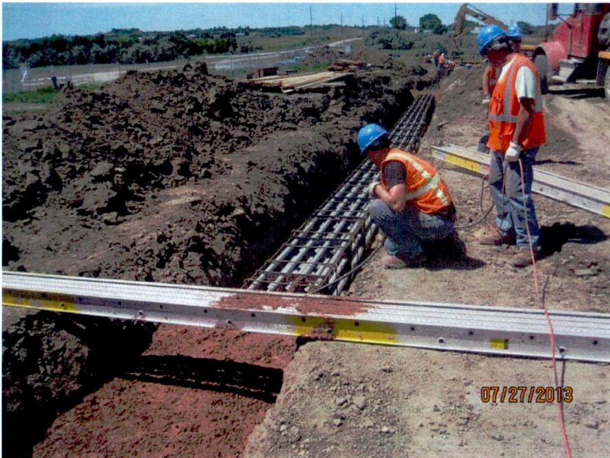
Duct bank concrete placement (looking W)
