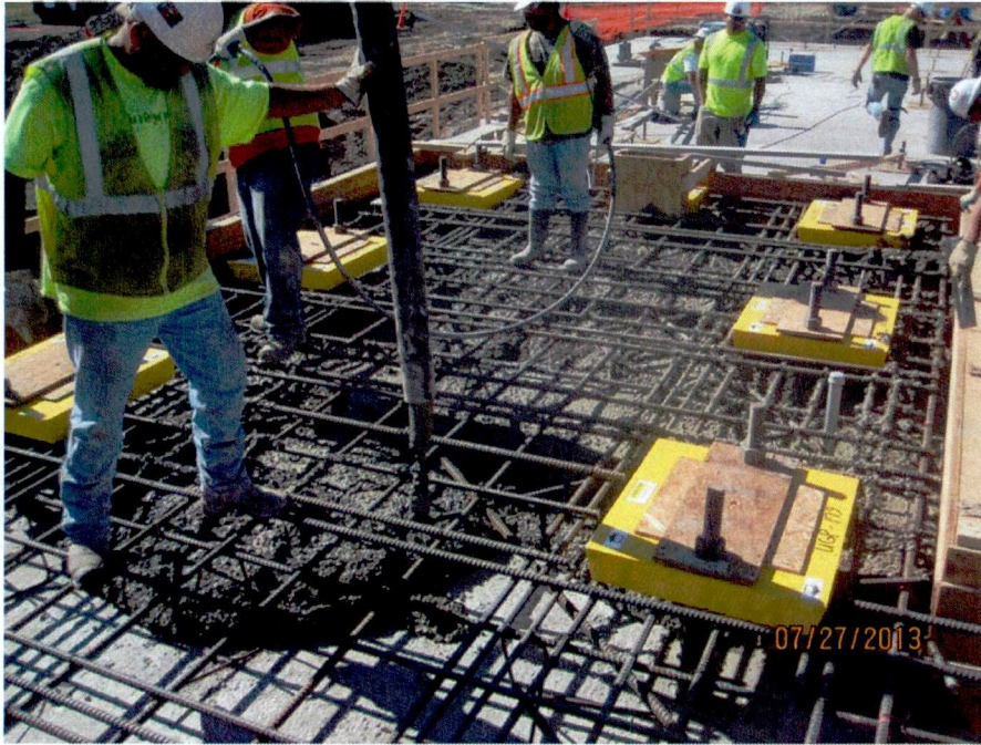
Generator pad concrete placement (looking S)
