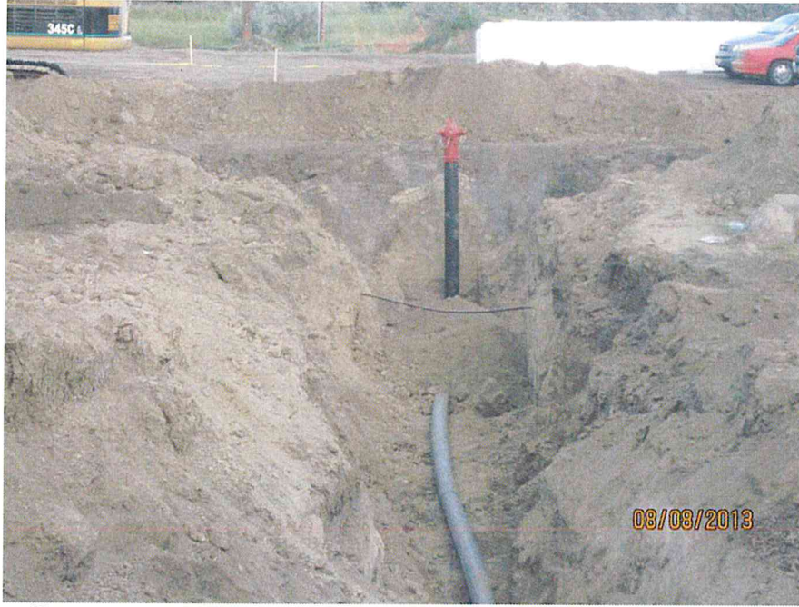
Fire protection piping and fire hydrant installation (looking W)
