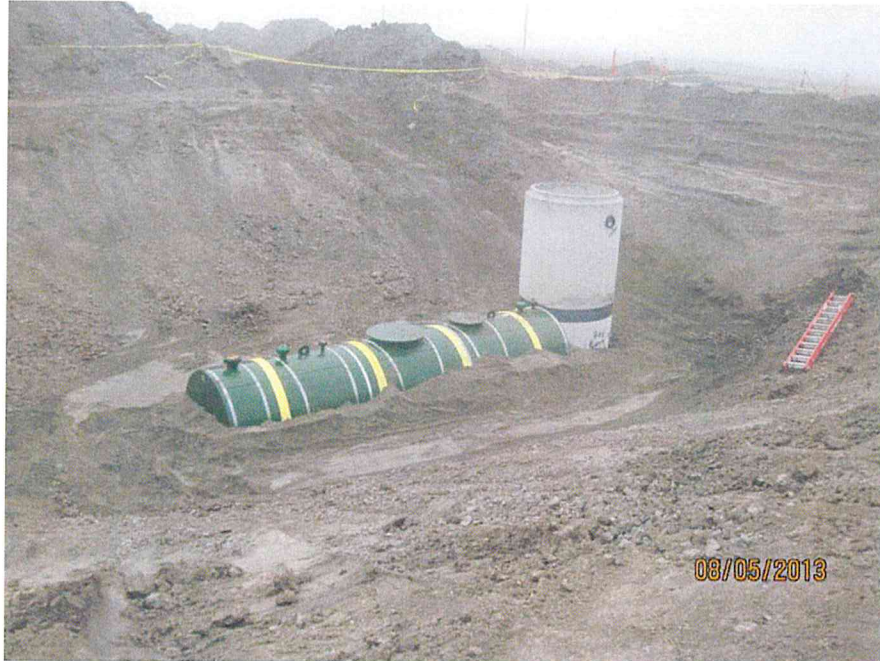
Emergency Oily Drain Tank and Lift Station manhole (looking SE)
