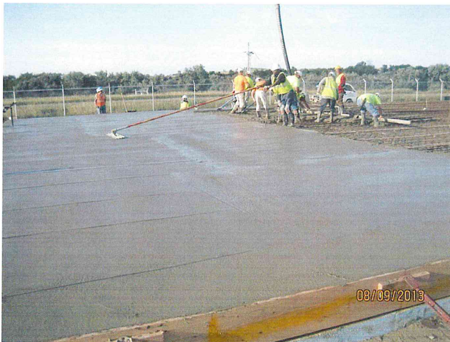
Service Building slab concrete placement (looking S)
