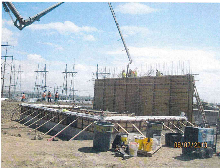
GSU pad and blast wall concrete placement (looking SE)
