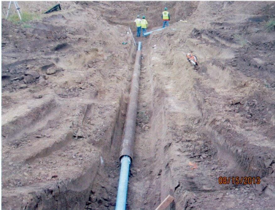
Wastewater force main installation (looking N)
