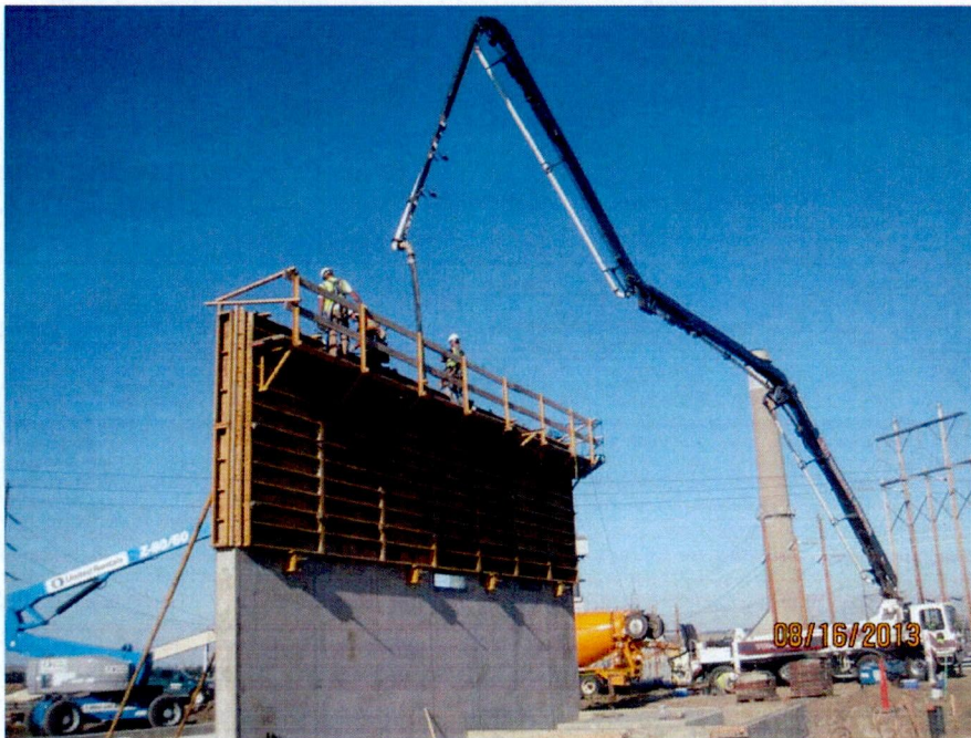
GSU blast wall concrete placement (looking NE)
