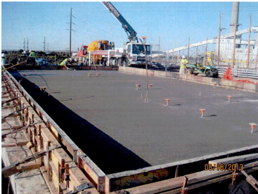
Closed cooling water module concrete placement (looking NE)
