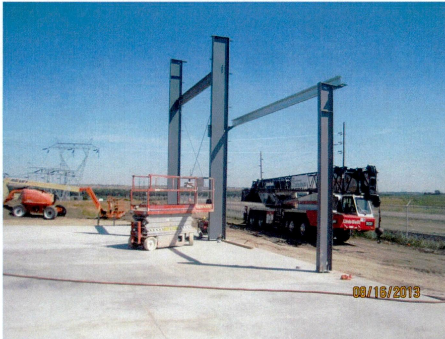
Service Building structural steel erection (looking E)
