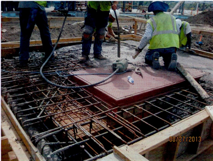
PEECC hatch concrete placement (looking SE)
