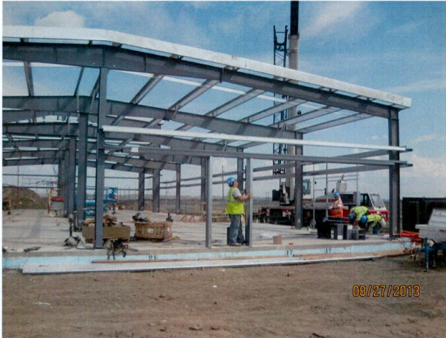
Service Building structural steel and door framing (looking E)
