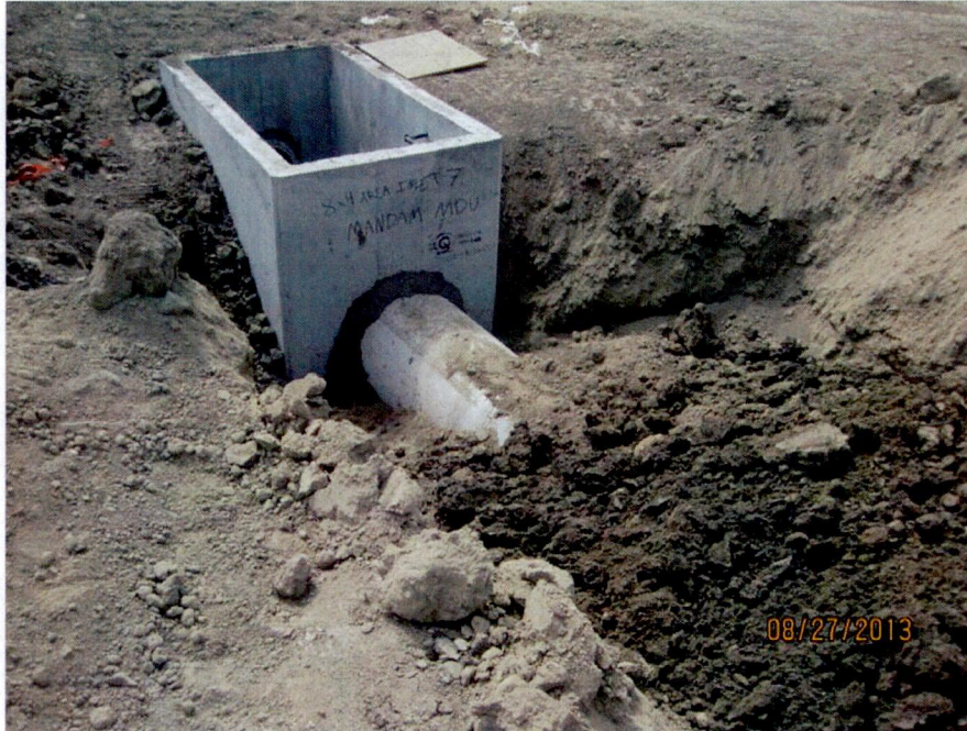
Stormwater structure installation (looking SW)
