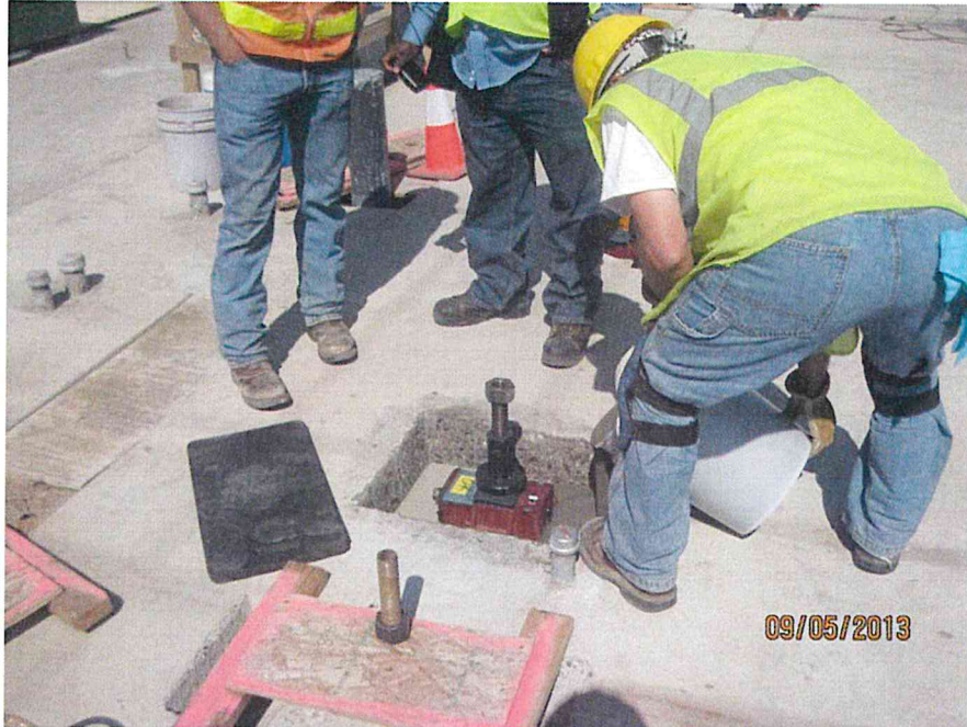
Turbine fixator grout installation (looking N)
