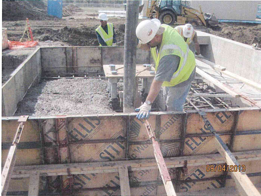
Inlet air filter concrete placement (looking S)
