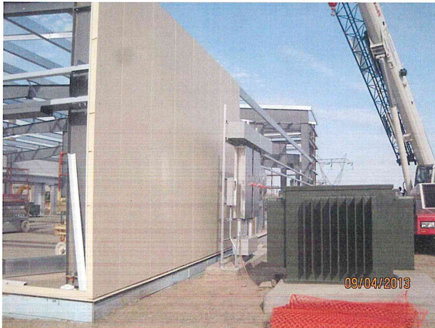
Service Building wall sheeting installation (looking E)
