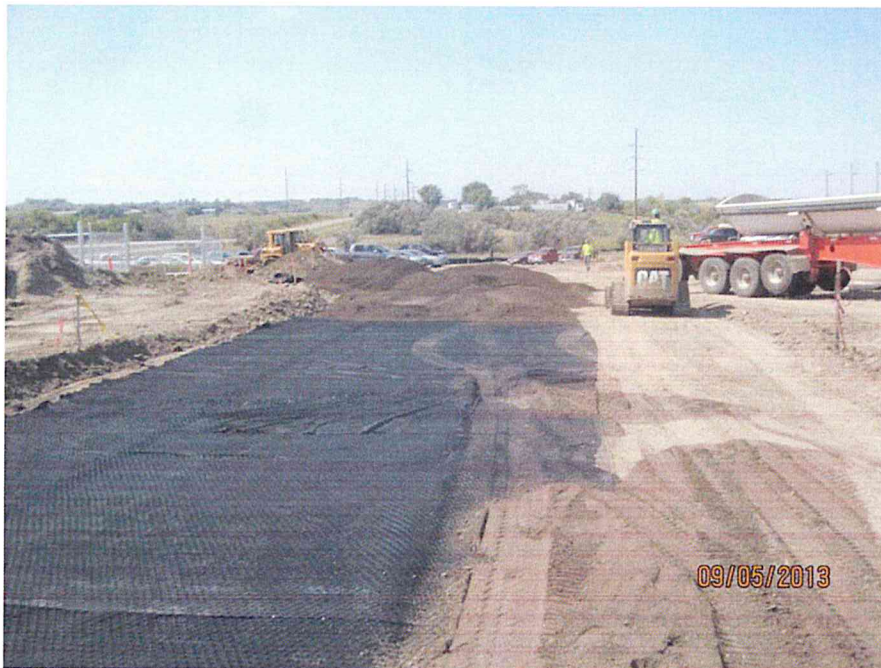
Heavy haul road Class 5 aggregate installation (looking W)
