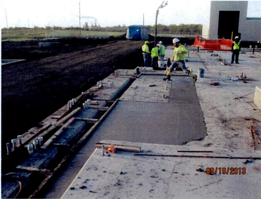
CT fill slab and trench drain concrete placement (looking S)
