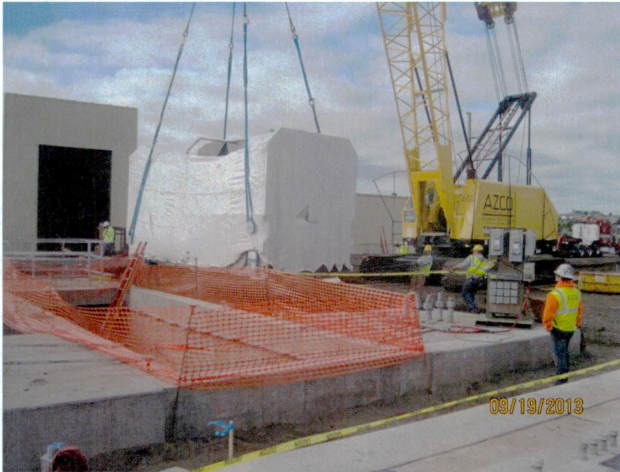
GE Turbine accessory base offloading (looking SW)
