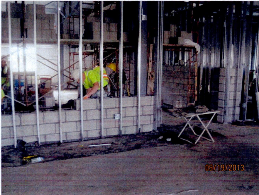
Service Building CMU wall installation (looking SW)
