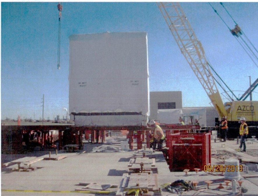
GE turbine jack and slide installation (looking S)
