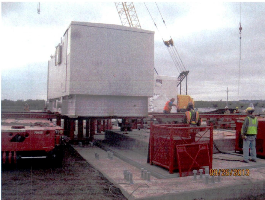
GE generator jack and slide installation (looking S)
