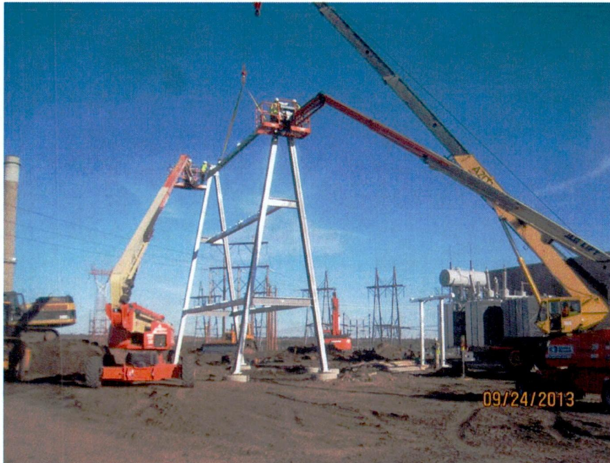
115kV A-frame structure installation (looking SE)
