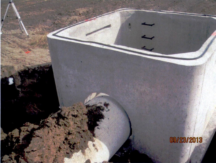
Stormwater basin outlet structure installation (looking NE)
