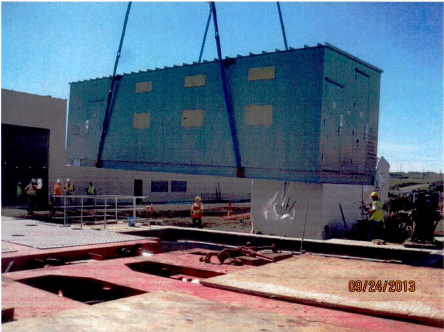
PEECC offloading and installation (looking SW)
