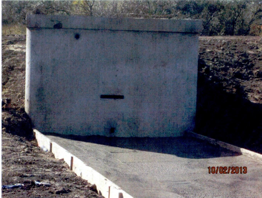
Stormwater basin trickle channel installation (looking W)
