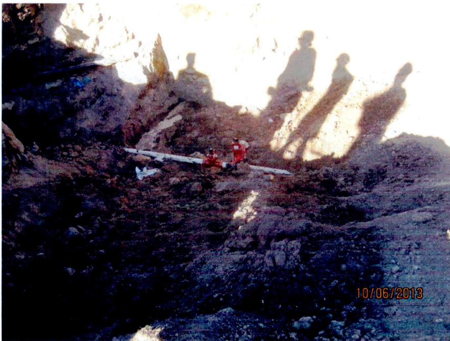
Service water valve installation (looking S)
