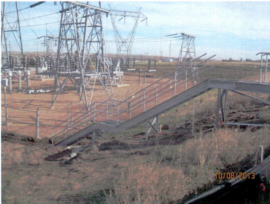
Steel access stairs installation (looking S)
