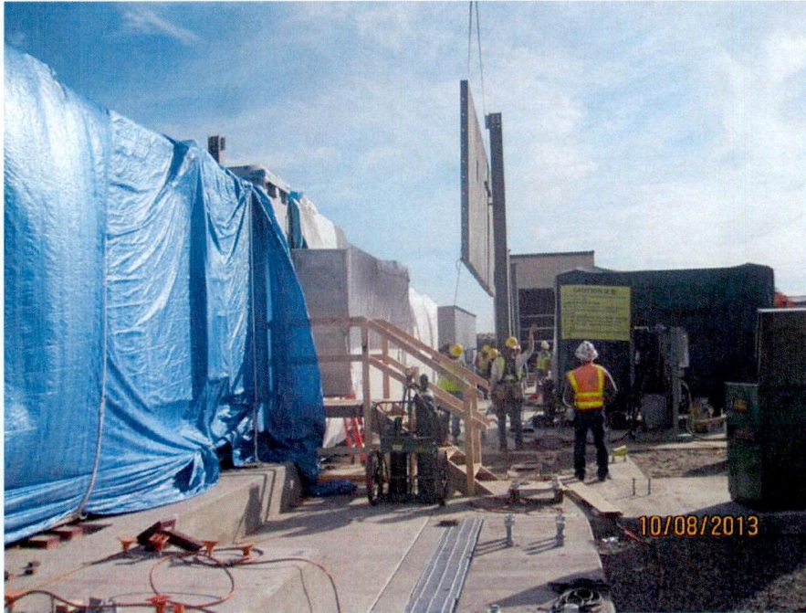
Accessory base enclosure wall installation (looking S)
