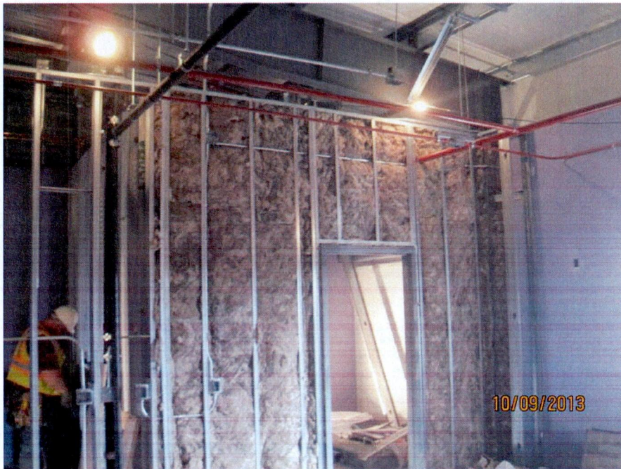
Service Building electrical, insulation, plumbing, and sheet rock installation (looking SW)
