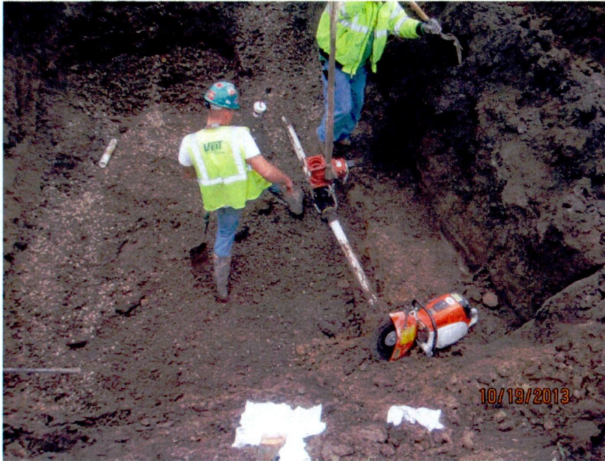
Service Building potable water isolation valve installation (looking SE)
