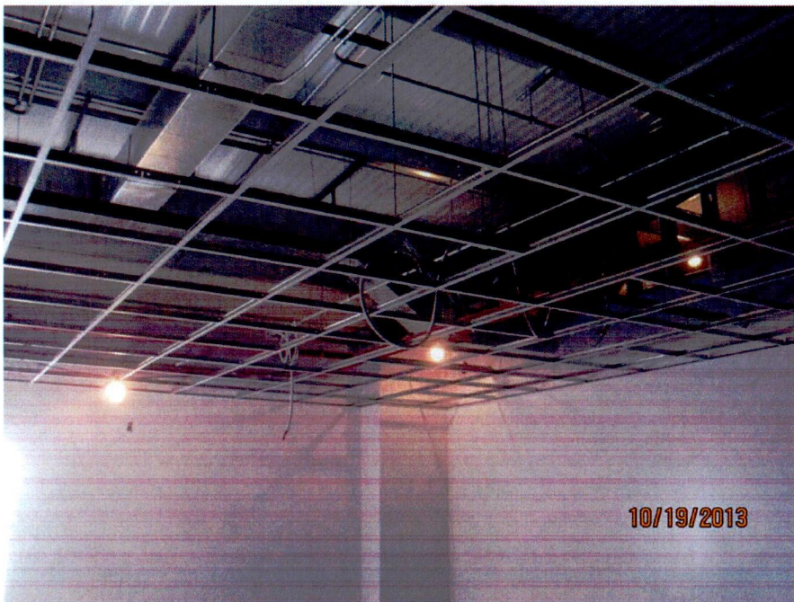
Service Building paint and drop ceiling installation (looking SW)
