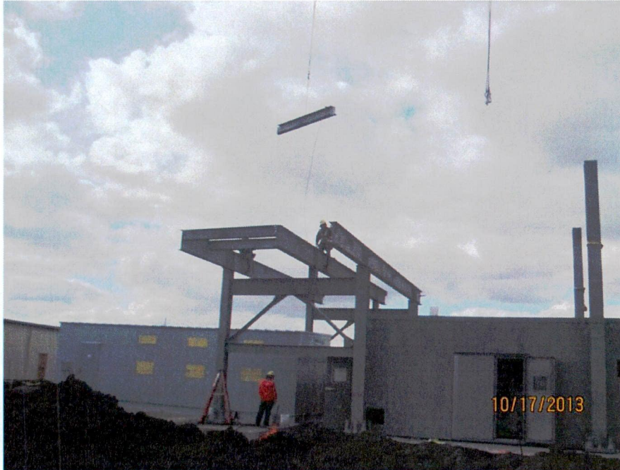
Inlet air filter structural steel erection (looking SW)
