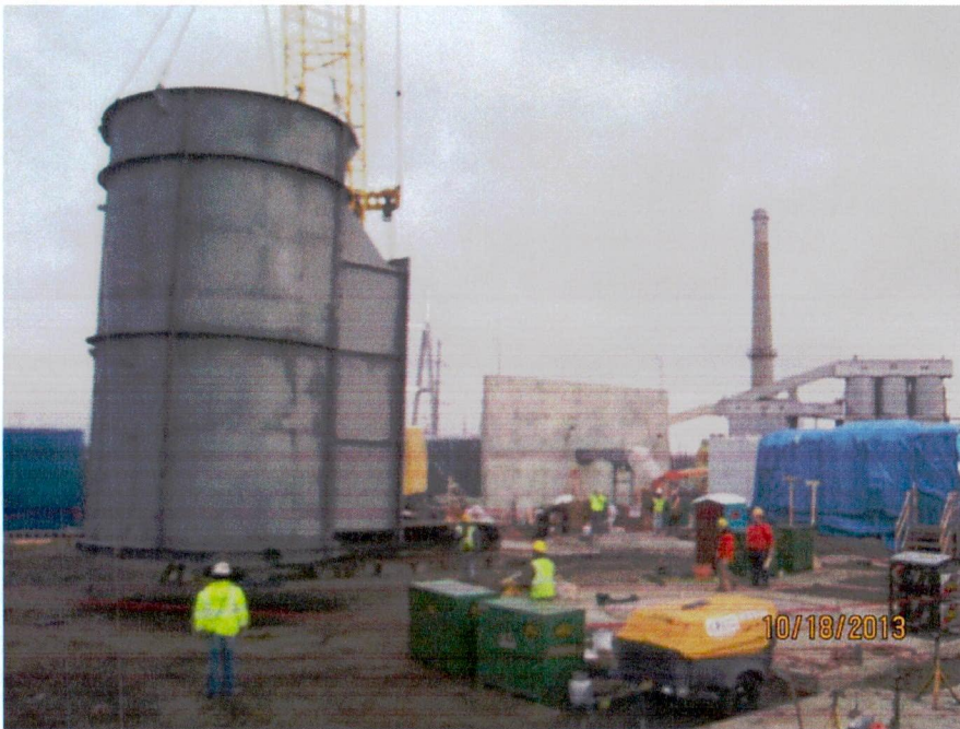
Lower section exhaust stack placement (looking NE)
