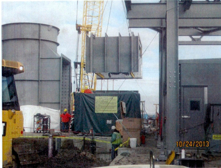
Exhaust system duct installation (looking N)
