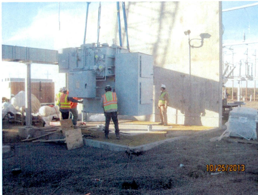
Unit Auxiliary Transformer (UAT) installation (looking NW)
