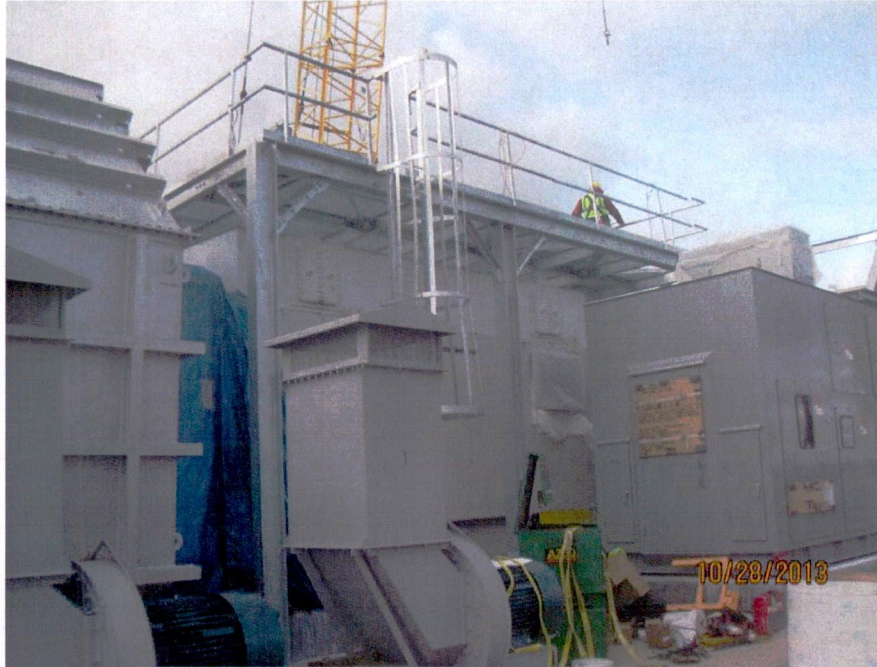
Generator platform installation (looking NW)
