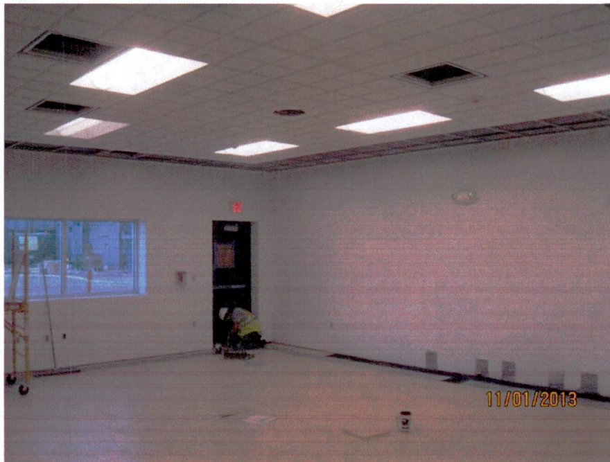
Service Building floor tile installation (looking NE)
