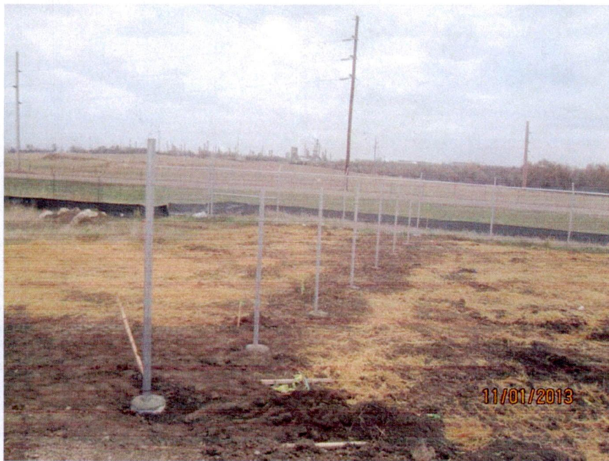
Site security fence installation (looking S)
