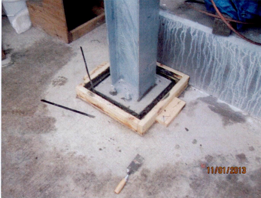
Generator platform base plate grout installation (looking SW)
