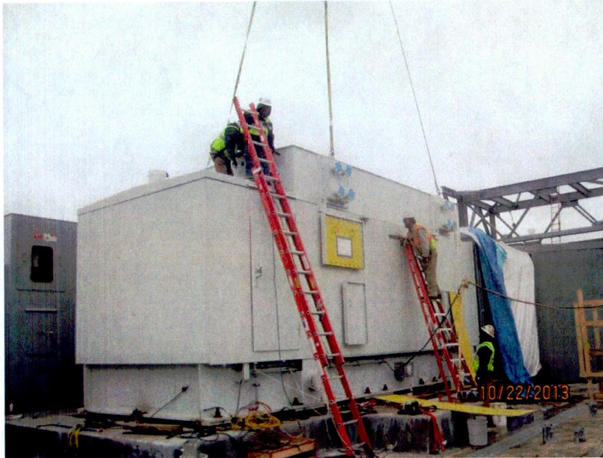
Generator heat exchanger installation (looking SE)
