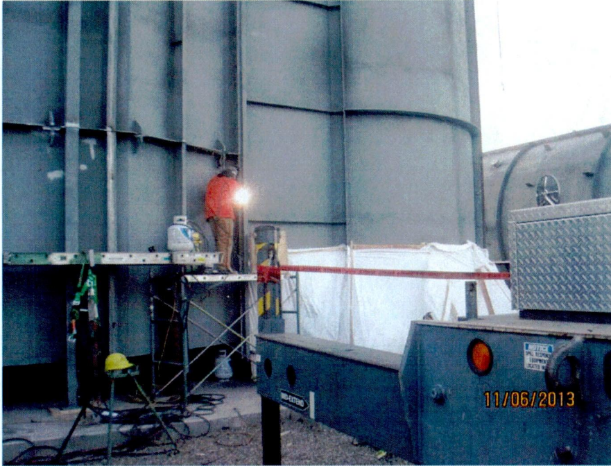
Exhaust stack installation (looking S)
