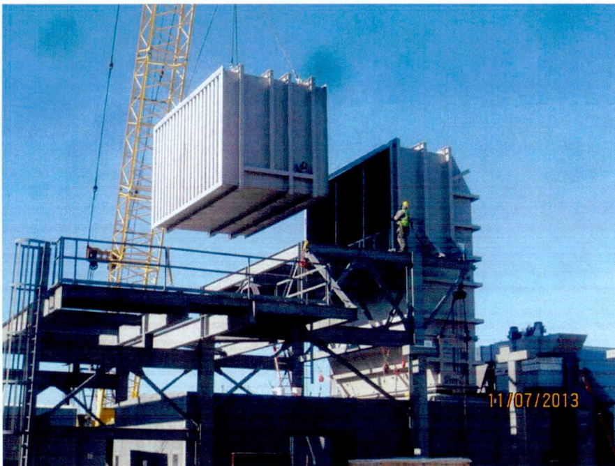
Inlet air filter installation (looking W)
