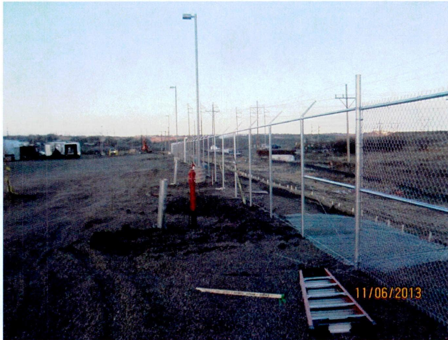
Site security fence installation (looking W)
