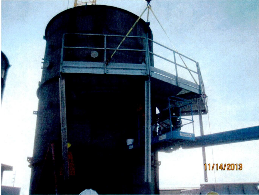
Exhaust stack platform installation (looking E)
