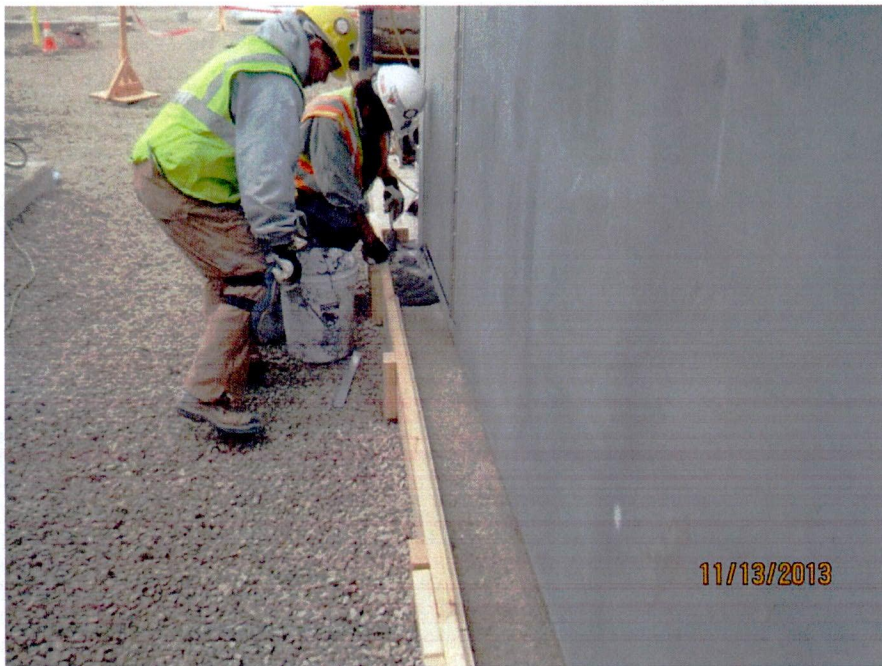
Accessory base enclosure grout installation (looking W)
