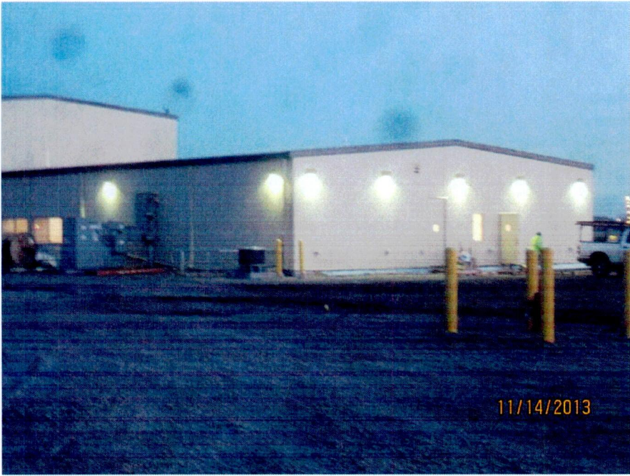
Service Building outside lights installation (looking SE)
