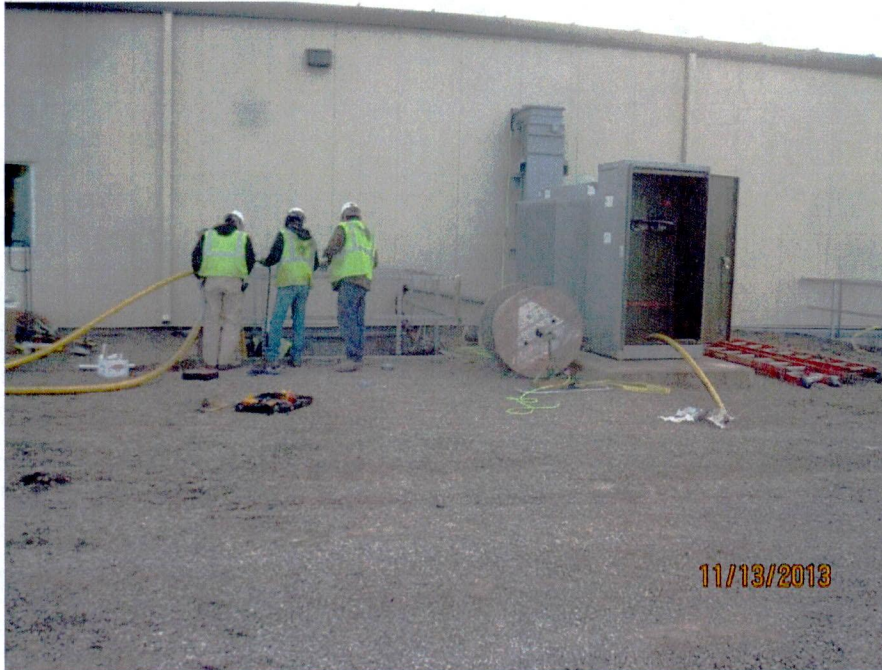
Cable installation (looking S)
