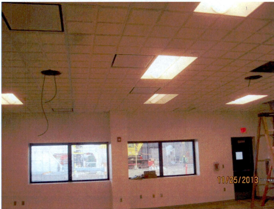
Service Building Gai-tronics installation (looking N)
