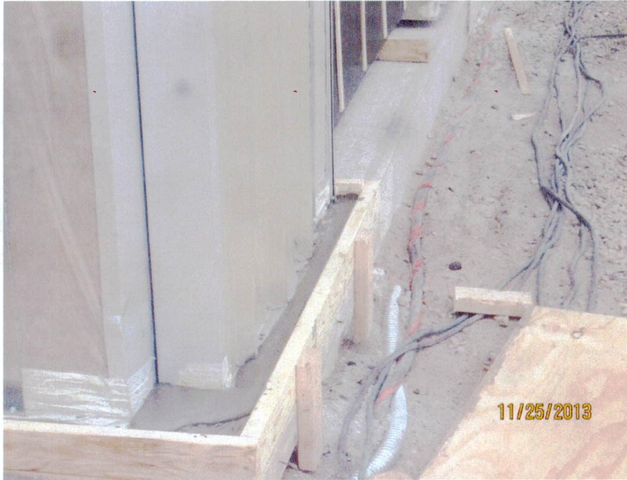
Accessory enclosure grout installation (looking N)
