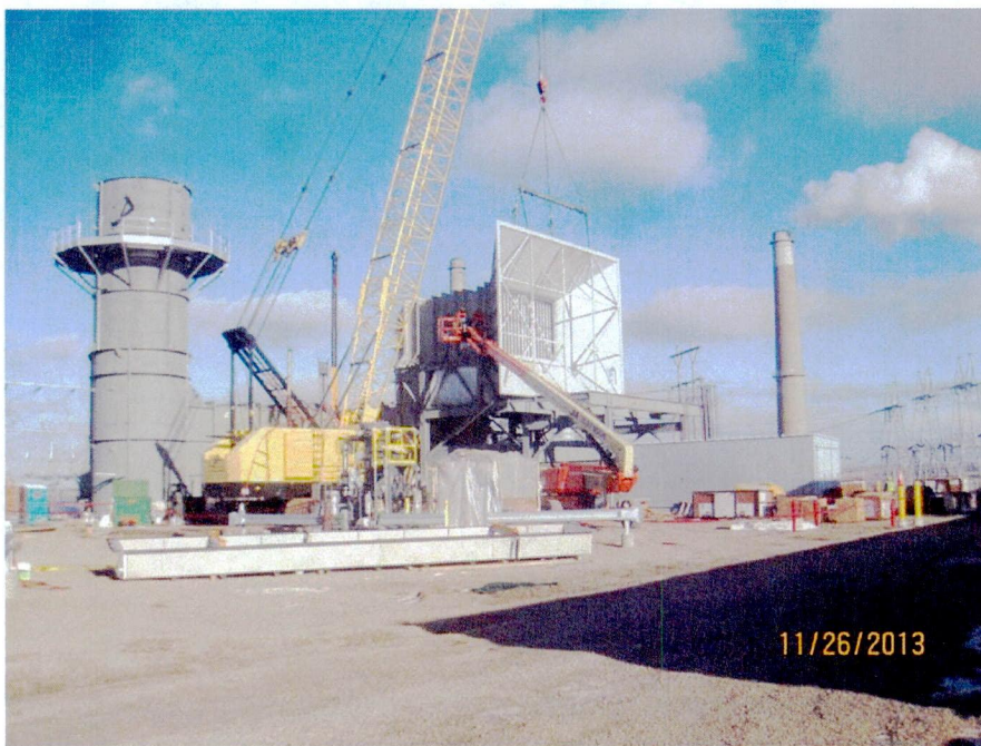
Inlet air transition section installation (looking NE)
