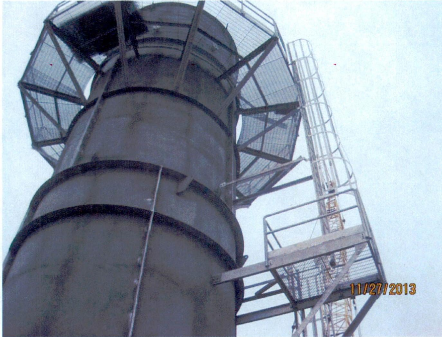
Exhaust stack ladder installation (looking S)
