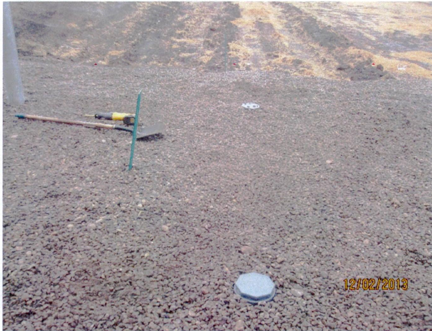
Septic tank inspection pipe cap installation (looking S)
