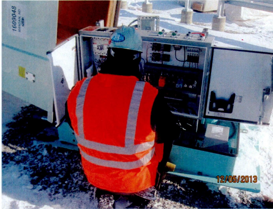
Wastewater lift station testing (looking E)
