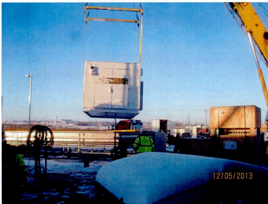
CEMS shelter installation (looking W)
