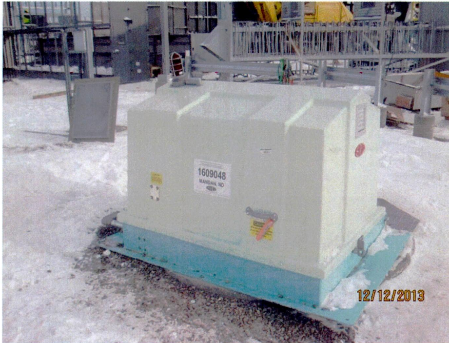
Lift station high level alarm light installation (looking NE)
