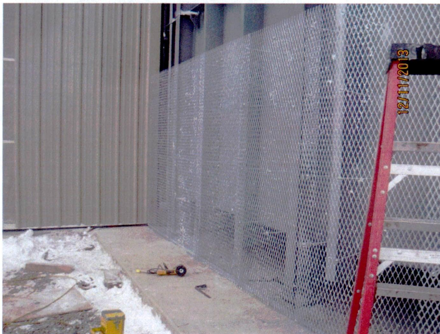
Exhaust stack personnel protection guard installation (looking E)
