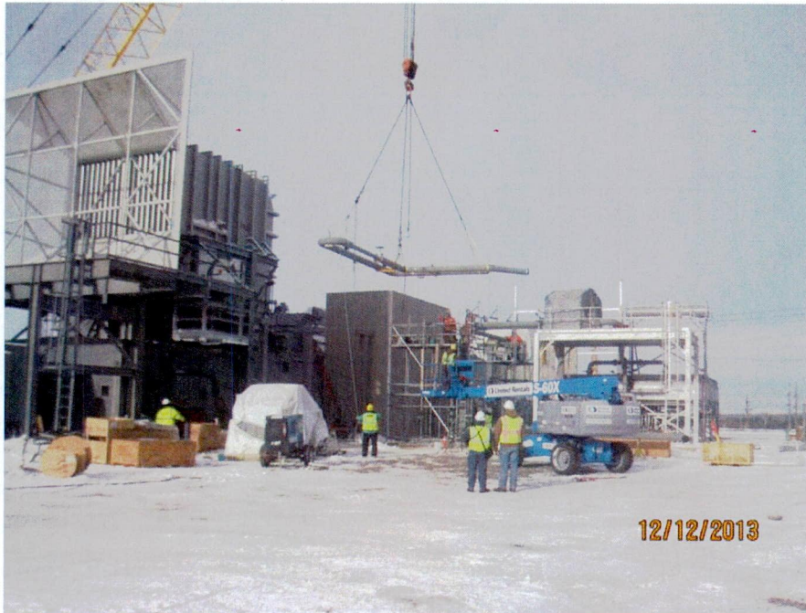
Closed cooling water loop installation (looking NW)
