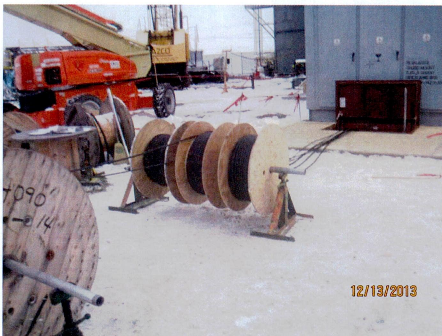
Cable pulling and installation (looking W)
