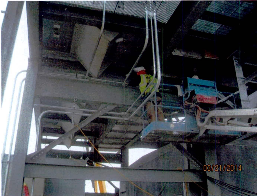
Inlet air filter conduit installation (looking W)
