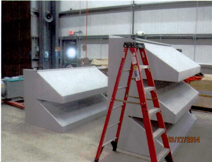
Inlet air filter louver fabrication (looking NE)
