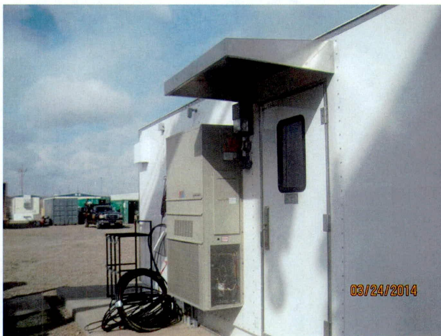
CEMS enclosure hook installation and light repair (looking NW)
