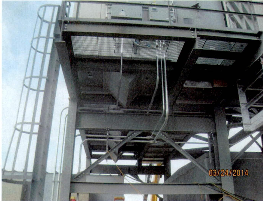
Air inlet filter conduit installation (looking W)
