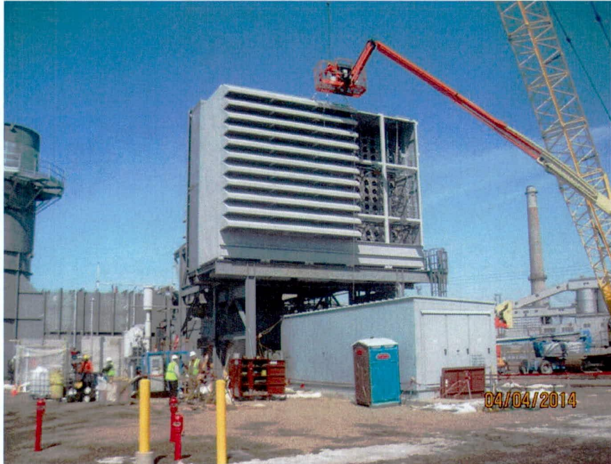
Air inlet filter louver installation (looking NE)
