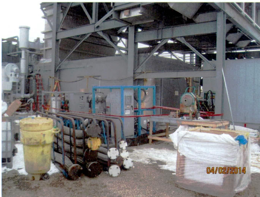
Lube oil preparation and flush (looking NE)
