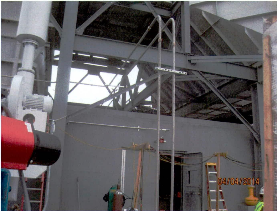
Water mist fire protection piping installation (looking E)
