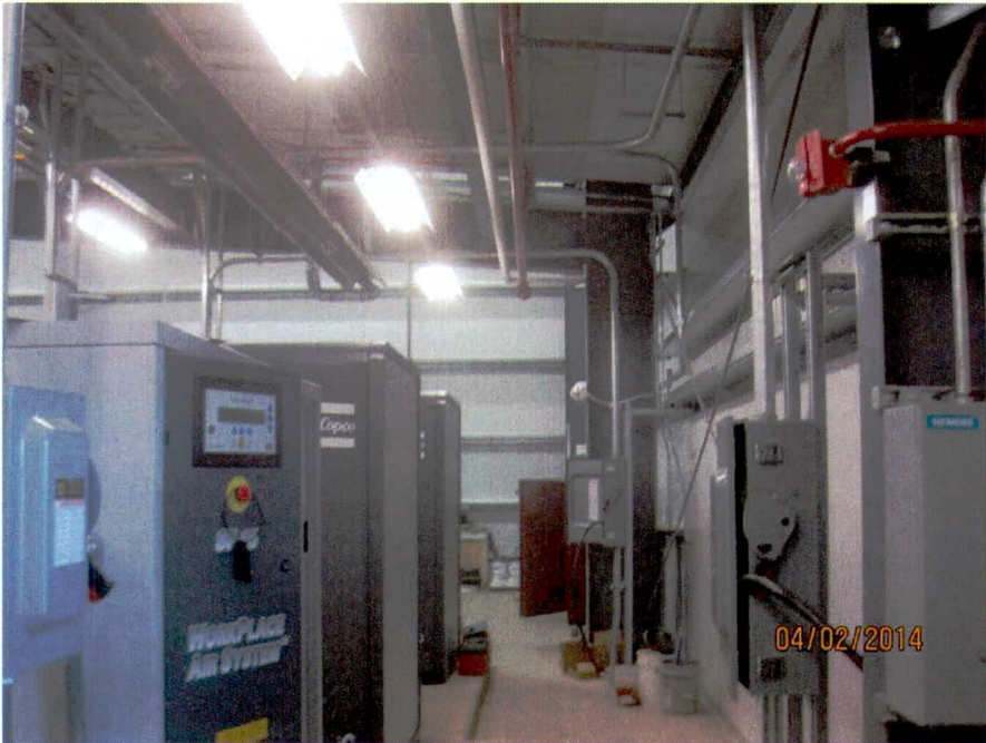
Air compressor disconnect switches and conduit installation (looking E)
