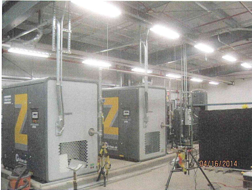
Air compressor piping installation (looking SW)
