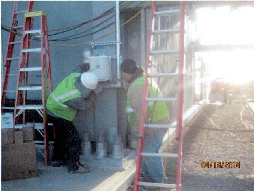
Gai-tronics box installation (looking E)
