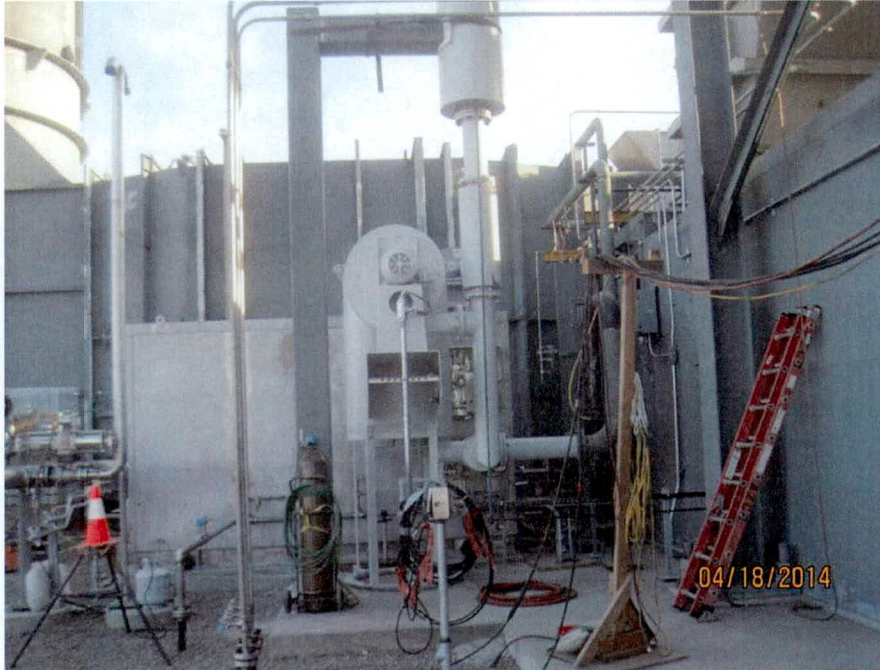
Oil mist eliminator support installation (looking N)
