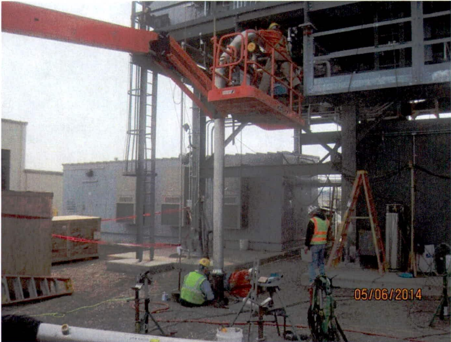
Evaporative cooler piping installation (looking W)
