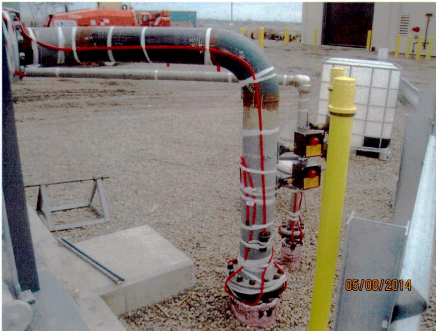
Fuel gas heat trace installation (looking S)
