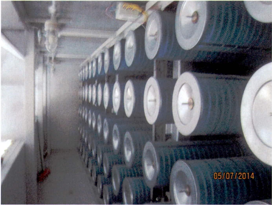
Inlet air filter installation (looking W)
