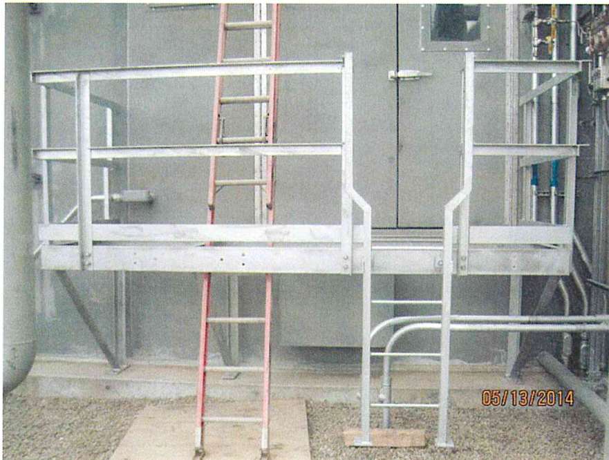
East turbine enclosure platform installation (looking W)
