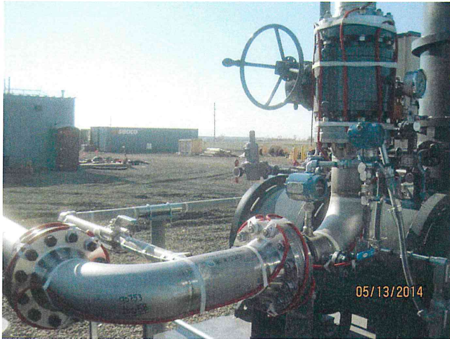
Fuel gas heat trace installation (looking SE)
