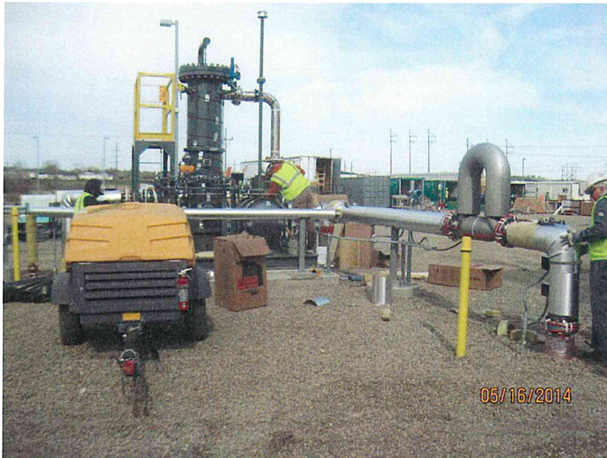
Fuel gas insulation installation (looking W)
