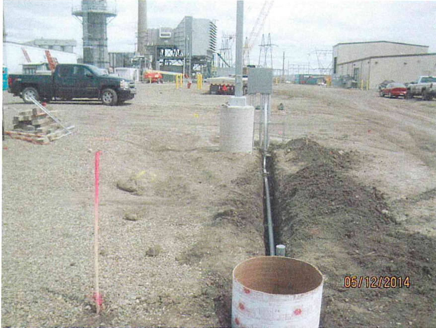
Card reader pedestal and conduit installation (looking E)
