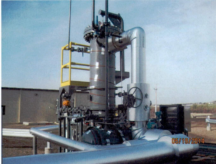
Coalescing filter heat trace installation (looking S)
