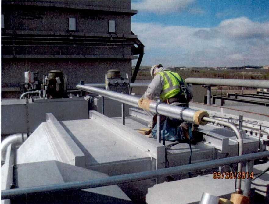
Piping insulation installation (looking SW)
