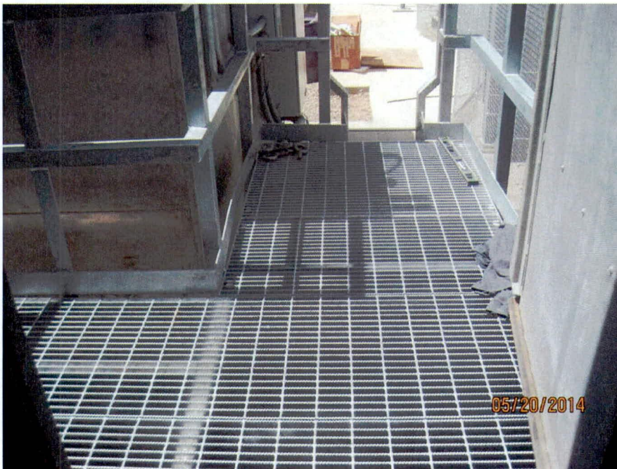
West turbine enclosure platform installation (looking W)
