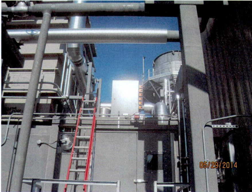
Instrument heated box installation (looking W)
