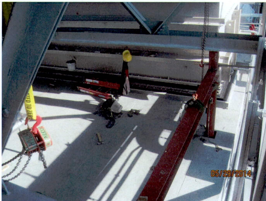
Accessory enclosure lifting beam installation (looking N)
