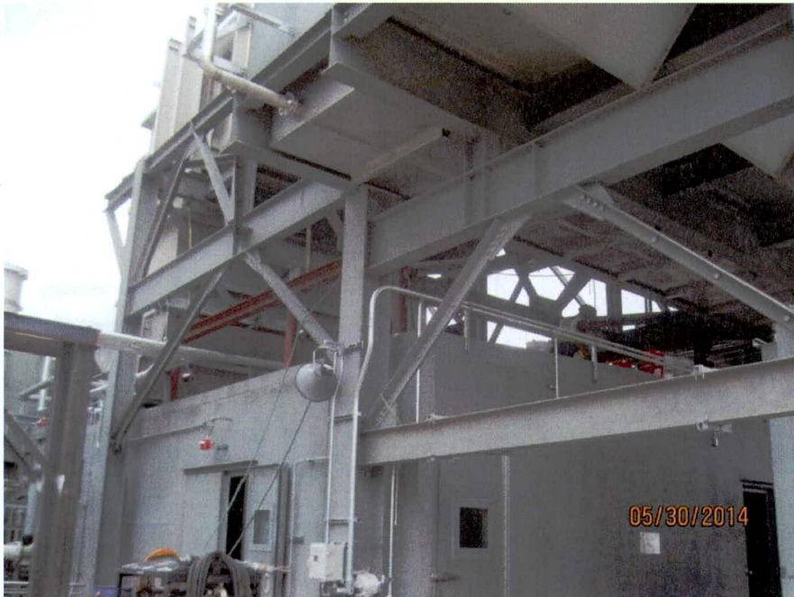
Accessory enclosure lifting beam installation (looking NE)
