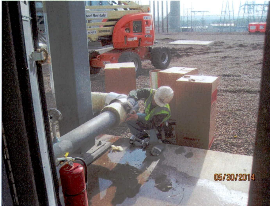
Piping insulation installation (looking E)
