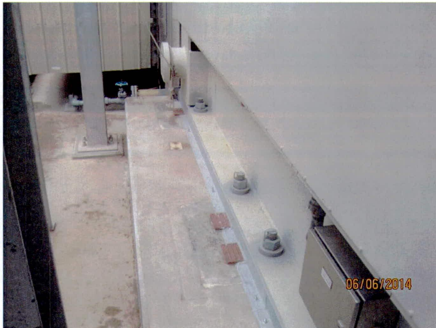
Generator trash guard installation (looking S)
