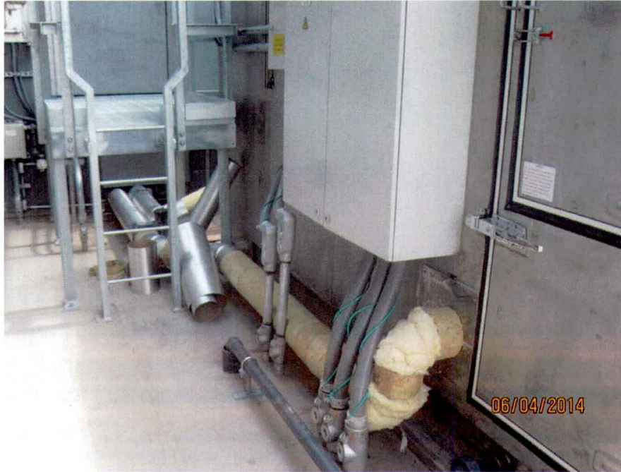
Fuel gas insulation installation (looking E)
