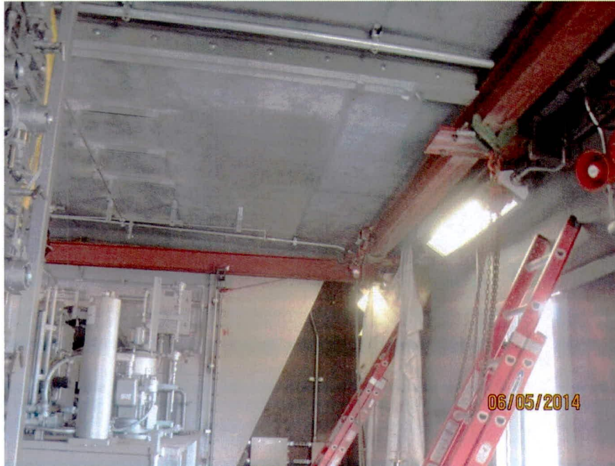
Accessory lifting system installation (looking N)
