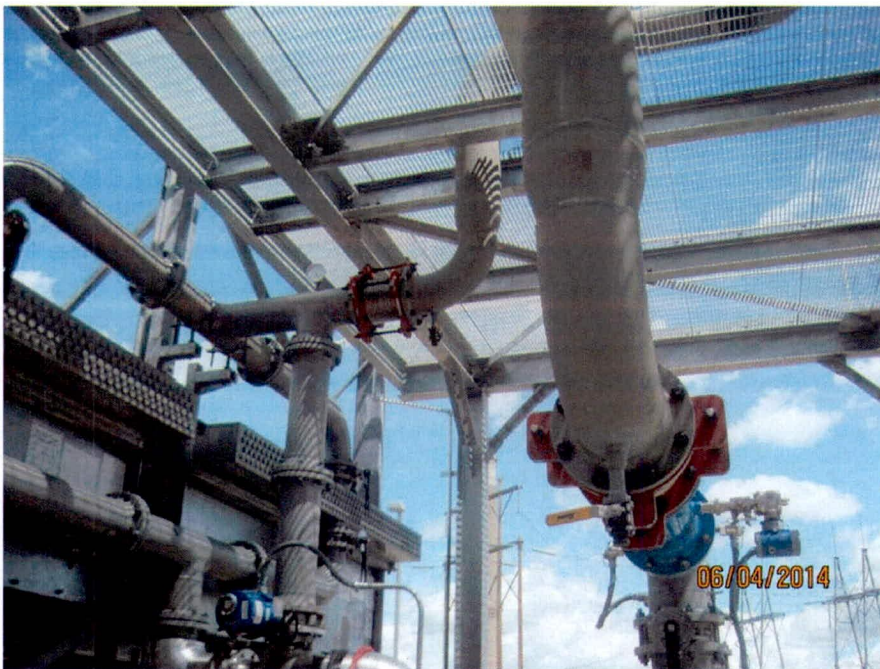
Cooling water expansion joint installation (looking E)
