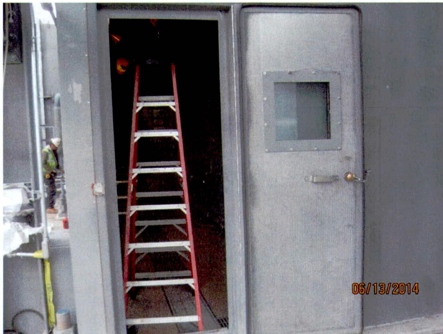
Enclosure door restraint installation (looking N)
