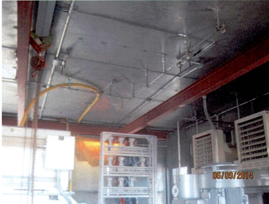
Accessory enclosure lifting beam installation (looking E)
