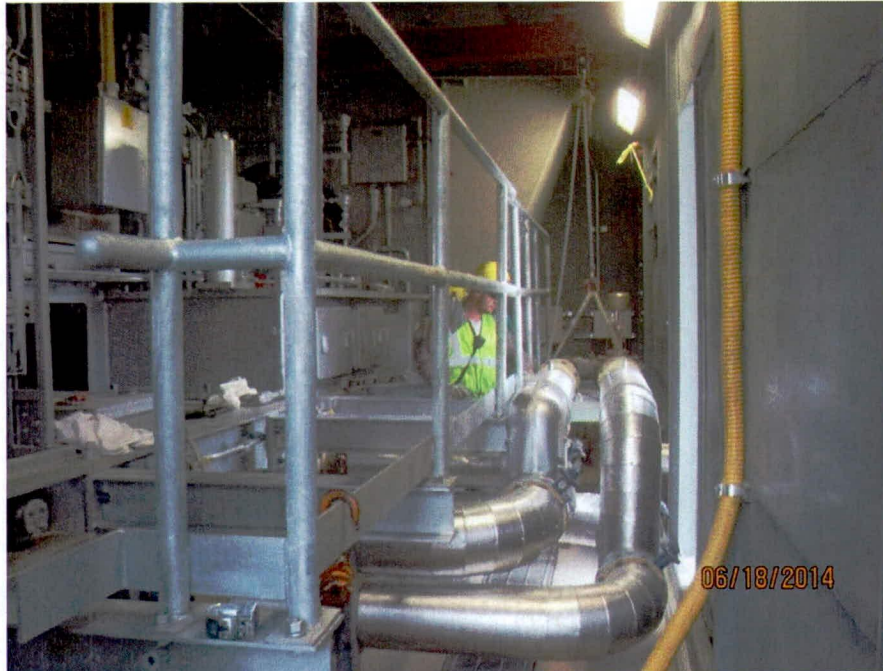
Accessory enclosure platform installation (looking N)
