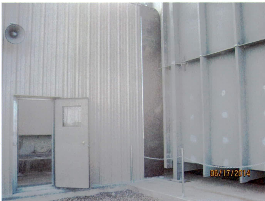
Acoustic wall gasket installation (looking E)
