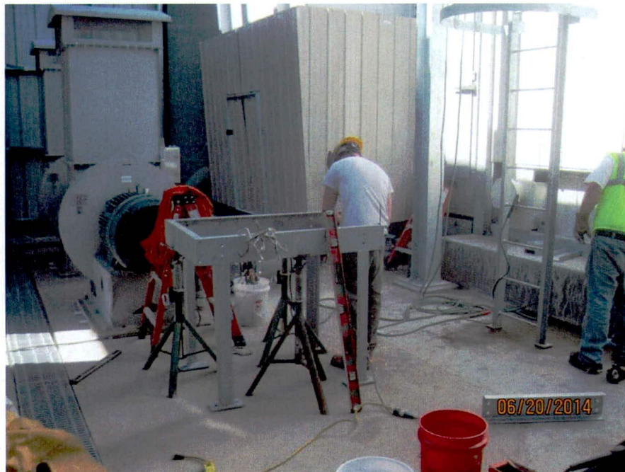
Generator access platform installation (looking SW)
