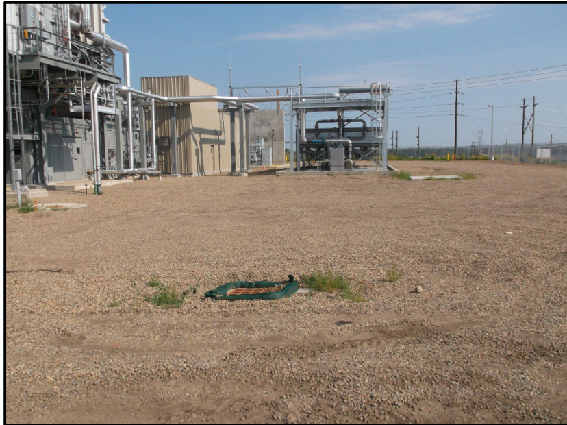
Photo 12. Direction: North. View of MDU 88 MW Combustion Turbine and stormwater inlet protection.
