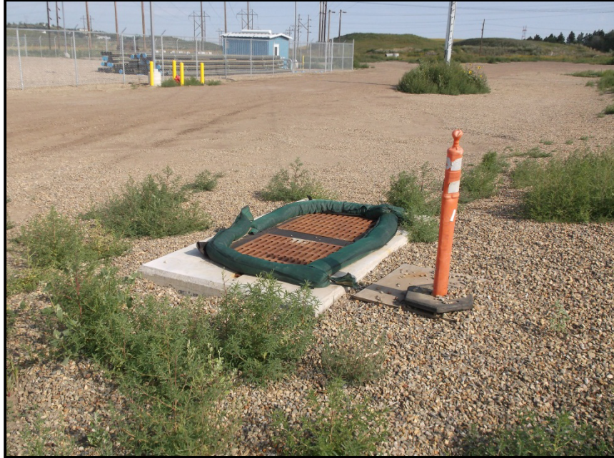
Photo 1. Direction: North. View of the stormwater inlet protection.
