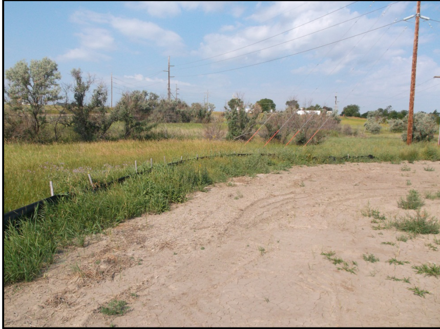
Photo 3. Direction: Northwest. View of silt fence along the project site boundary.
