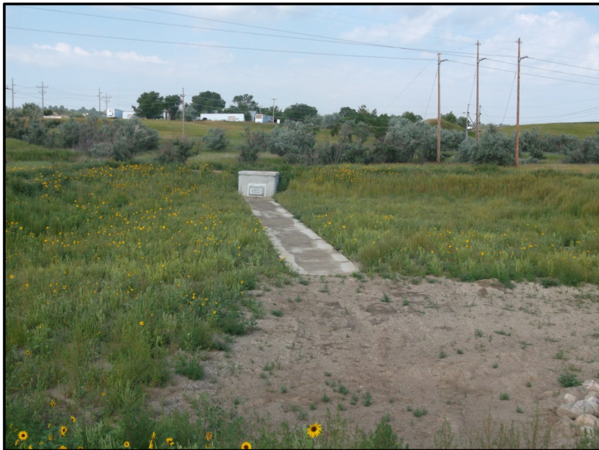
Photo 4. Direction: West. View of the drainage basin and valley gutter. Also pictured is the part of the finished stormwater pond.
