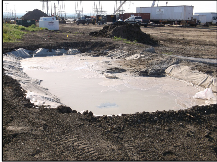
Photo 15. Direction: East. View of concrete washout pit, with liner, during construction.
