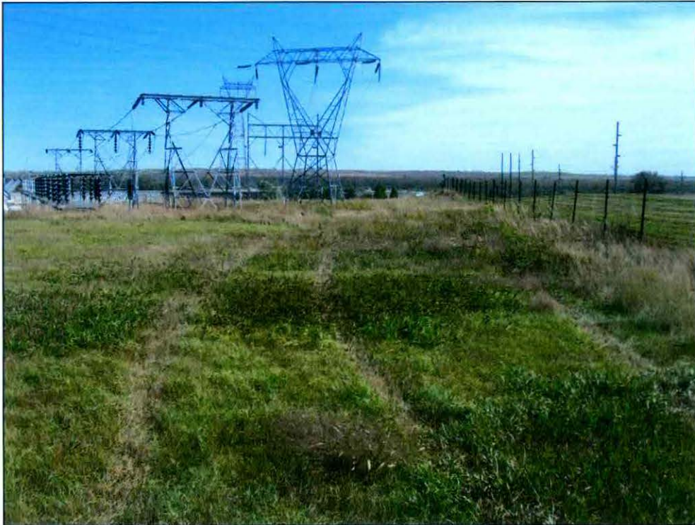
Figure 2: Overview of project area, view to the east.
