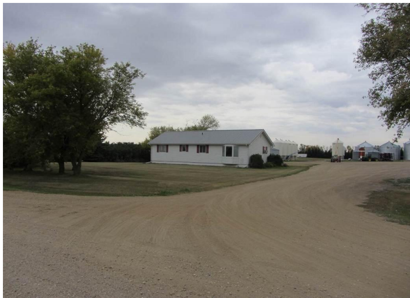
Photograph 3. A view of architectural feature 1 (with features 2 and 4 in the background) from 184th St NE. Photograph looking SW.
