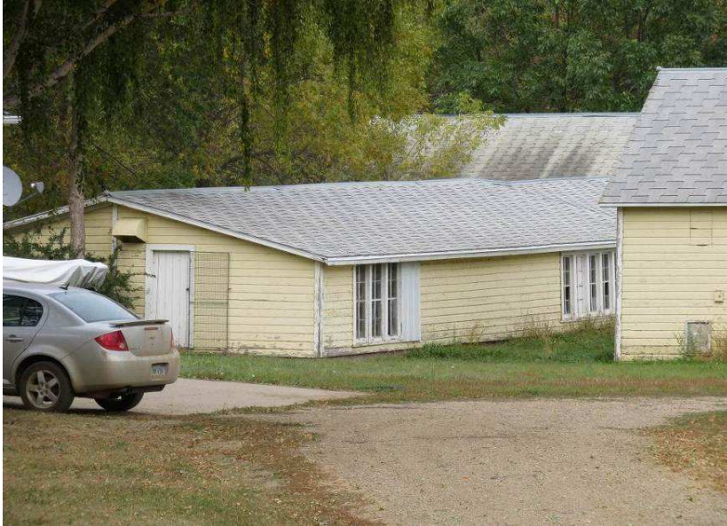
Photograph 7. A view of architectural feature 2 from 158th St NE from west of the farm. Photograph looking NE.
