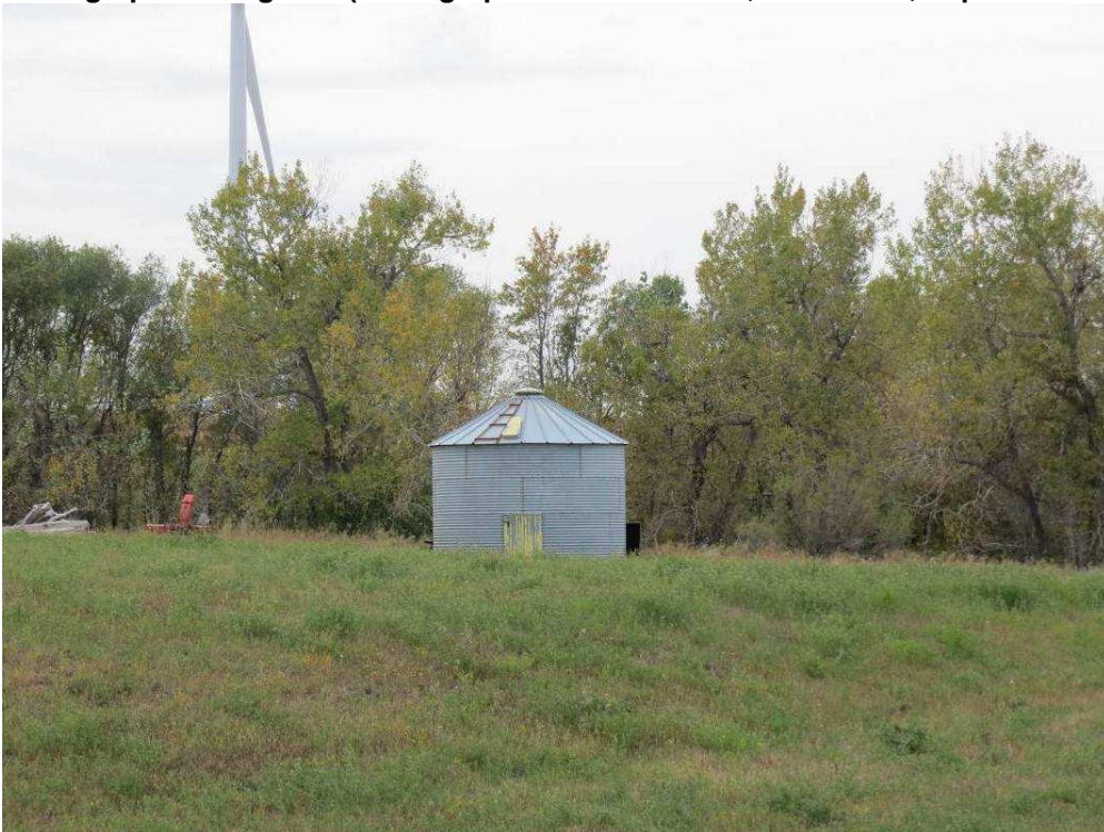
Photograph 94. A view of architectural feature 1 from 158th ST NE from east of the farm. Photograph looking W. (Photographer: Adam Holven, Tetra Tech, September 20, 2012.)
