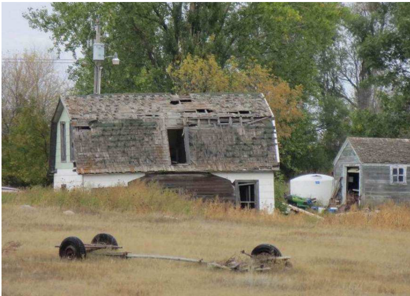
Photograph 10. A view of the former residence from 158th St NE from south of the farm. Photograph looking NNE.
