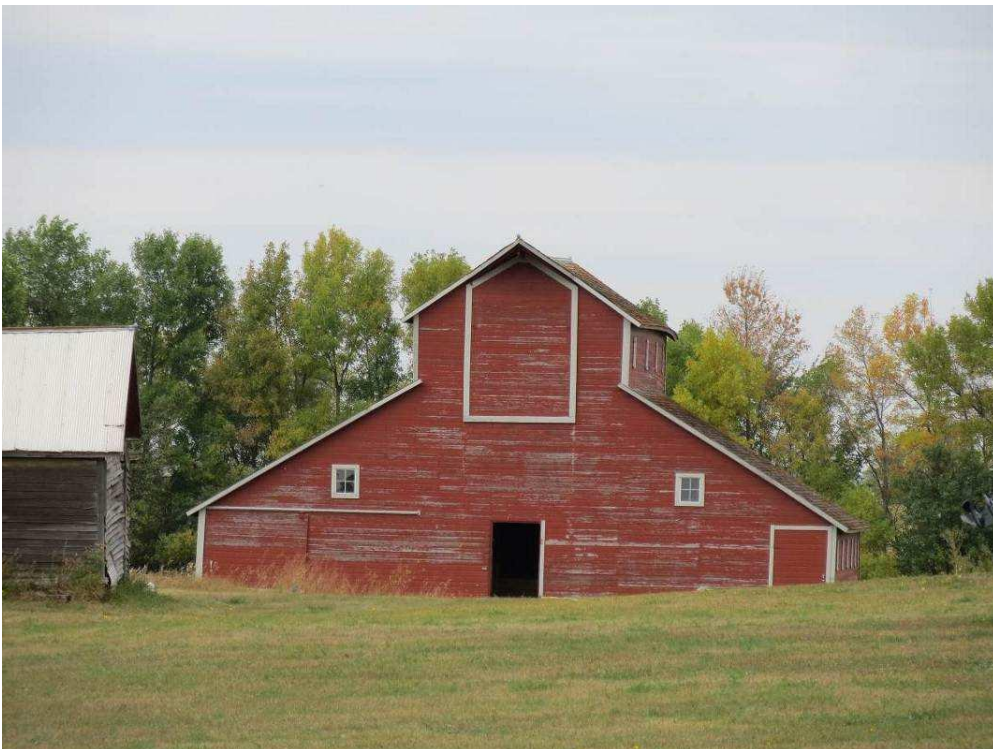
Photograph 13. A view of architectural feature 9 from the south along 279th Ave NE. Photograph looking N. (Photographer: Adam Holven, Tetra Tech, September 20, 2012.)
