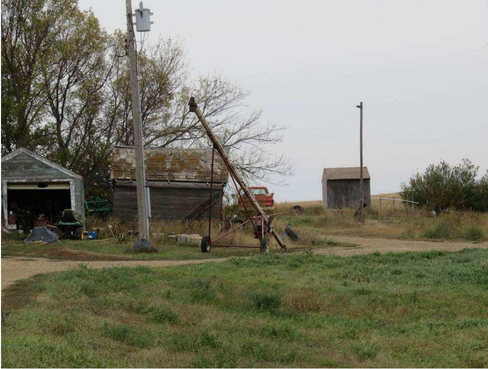
Photograph 76. A view (from left to right) of architectural features 9, 8, and 10 from 158th St NE from west of the farm. Photograph looking E. (Photographer: Adam Holven, Tetra Tech, September 20, 2012.)
