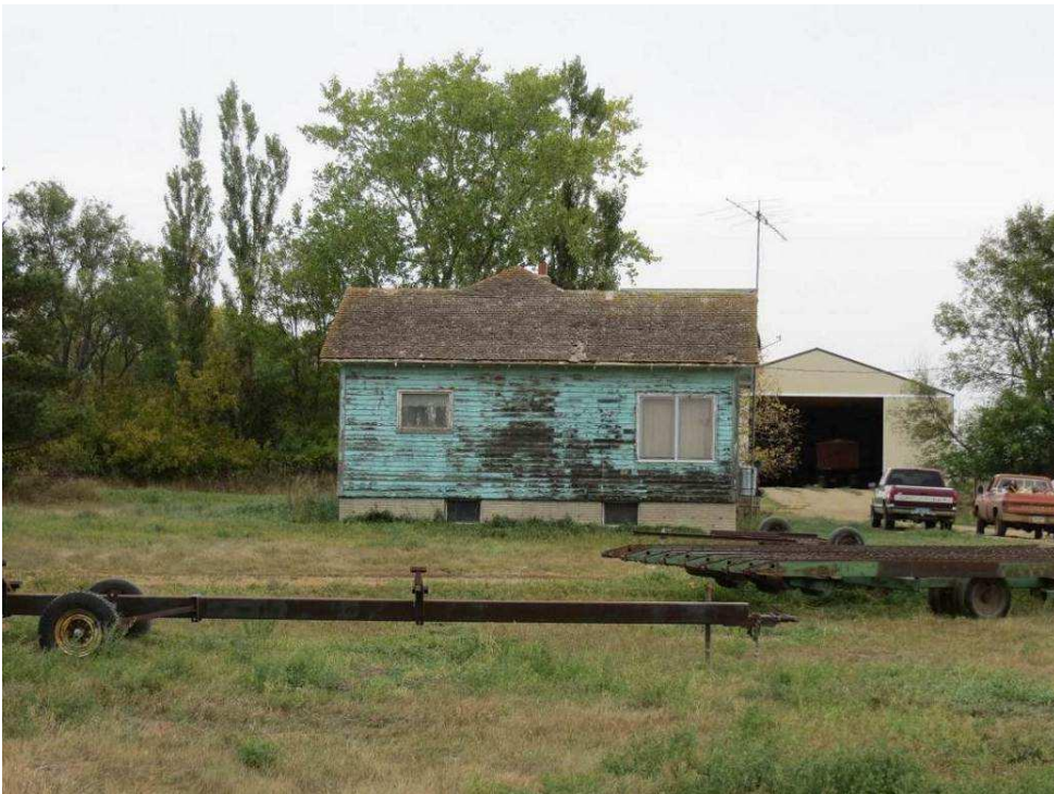
Photograph 67. A view of architectural features 1 and 2 from 158th St NE west of the farm. Photograph looking E. (Photographer: Adam Holven, Tetra Tech, September 20, 2012.)
