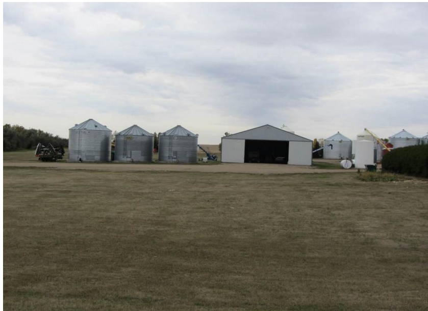
Photograph 5. A view of architectural features 2, 3, and 4 (left to right) from 184th St NE. Photograph looking W.
