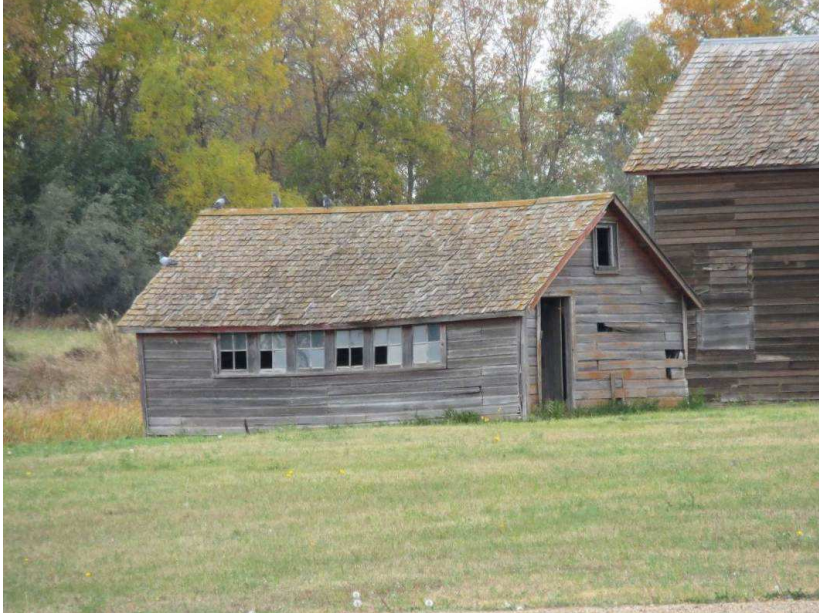
Photograph 9. A view of architectural feature 7 from the south along 279th Ave NE. Photograph looking NW.
