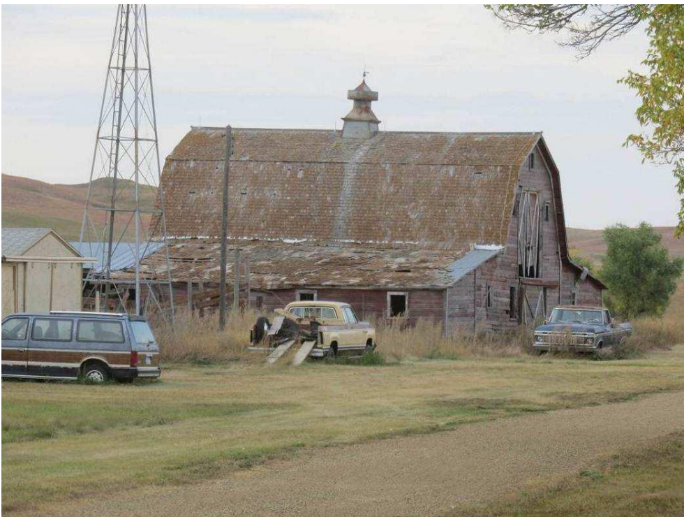
Photograph 41. A view of architectural feature 2 from 240th Ave NE. Photograph looking NNW. (Photographer: Adam Holven, Tetra Tech, September 20, 2012.)
