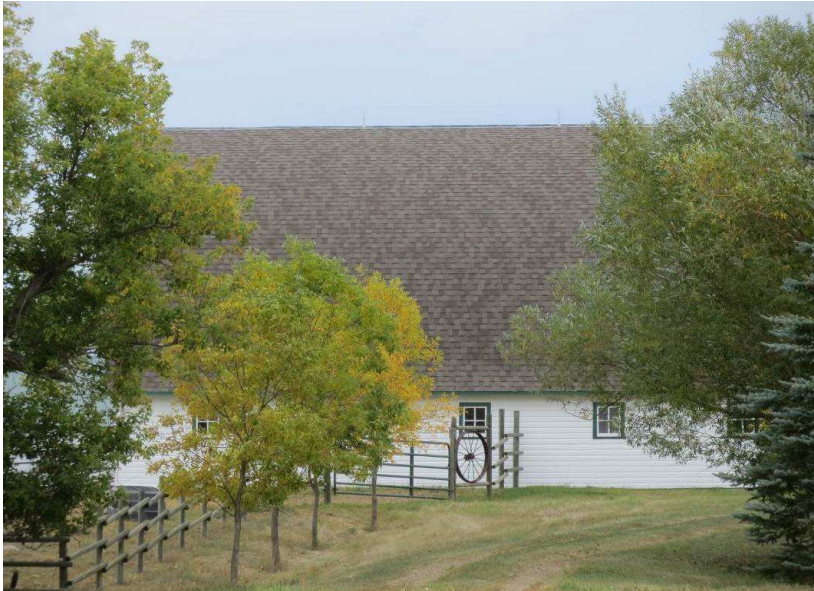
Photograph 9. A view of architectural feature 3 from 171st St NE. Photograph looking E.
