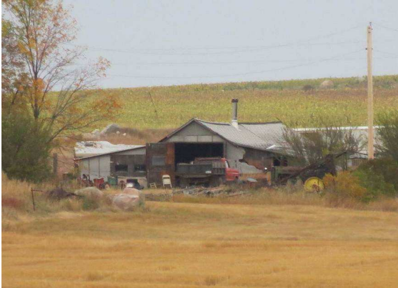
Photograph 3. A view of architectural feature 1 from 26th St NE from west of the farm. Photograph looking E-NE.
