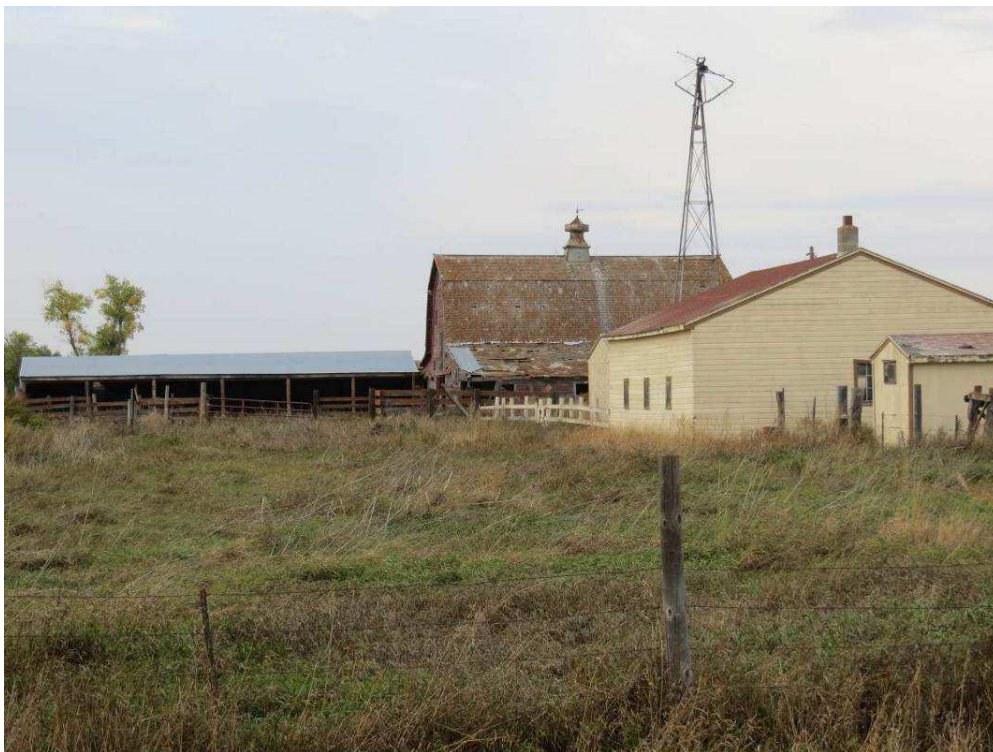
Photograph 35. A view of the west side of F5 from 240th Ave NE. Photograph looking N. (Photographer: Adam Holven, Tetra Tech, September 20, 2012.)
