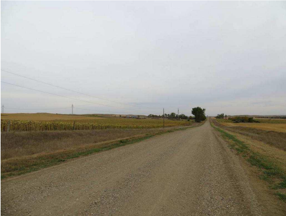
Photograph 60. A view of F7 from 158th St NE from north of the farm. Photograph looking SSE. (Photographer: Adam Holven, Tetra Tech, September 20, 2012.)
