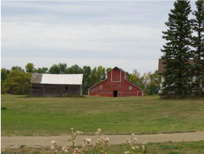
Photograph 11. A view of architectural feature 6 (right) and architectural feature 9 (left) from the south along 279th Ave NE. Photograph looking N.
