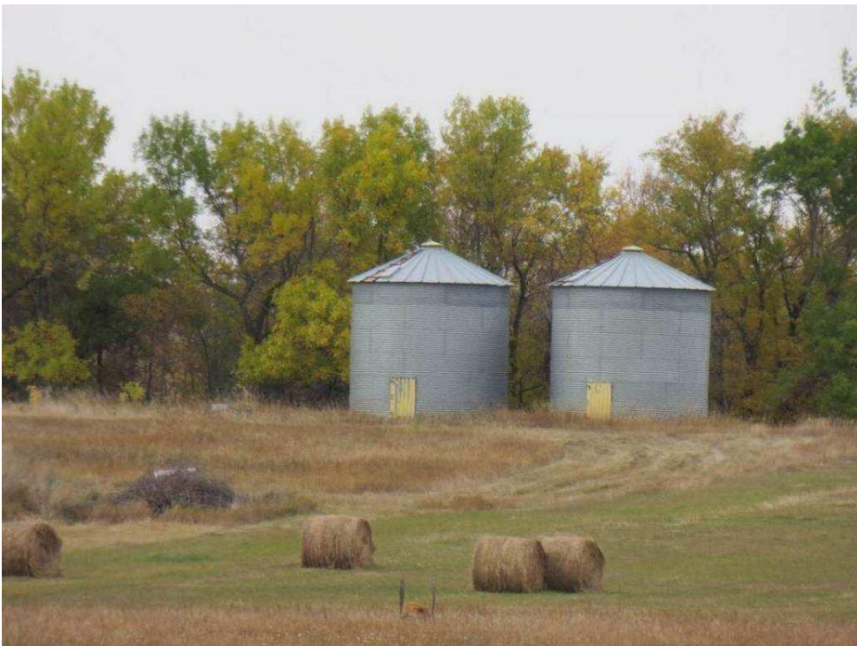
Photograph 107. A view of architectural feature 6 from 266th Ave NE from south of the farm. Photograph looking NNW. (Photographer: Adam Holven, Tetra Tech, September 20, 2012.)
