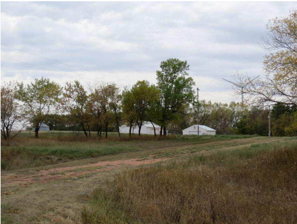
Photograph 90. A view (from left to right) of architectural features 1, 2, and 3 from 158th St NE from northeast of the farm. Photograph looking SW. (Photographer: Adam Holven, Tetra Tech, September 20, 2012)
