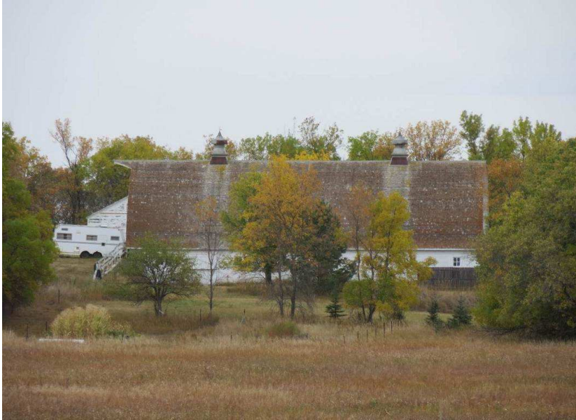
Photograph 11. A view of architectural feature 4 from 266th Ave NE, south of the farm. Photograph looking N-NW.
