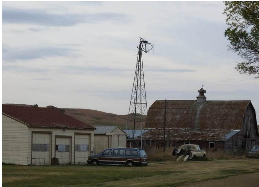
Photograph 13. A view of architectural features 11, 10, 16, and 9 (left to right) from 240th Ave NE. Photograph looking NNW.
