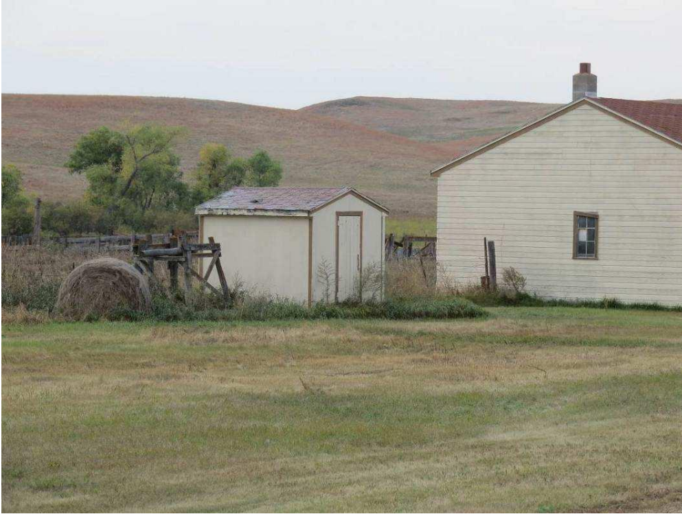
Photograph 44. A view of architectural feature 14 (left) and 11 from 240th Ave NE. Photograph looking NW. (Photographer: Adam Holven, Tetra Tech, September 20, 2012.)
