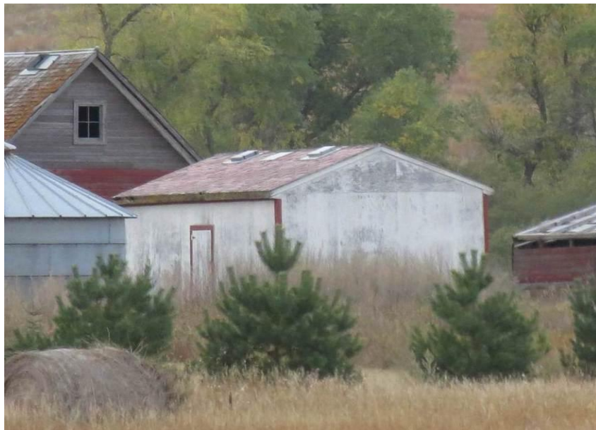
Photograph 21. A view of architectural feature 6 from 240th Ave NE and 171st St NE. Photograph looking NW.
