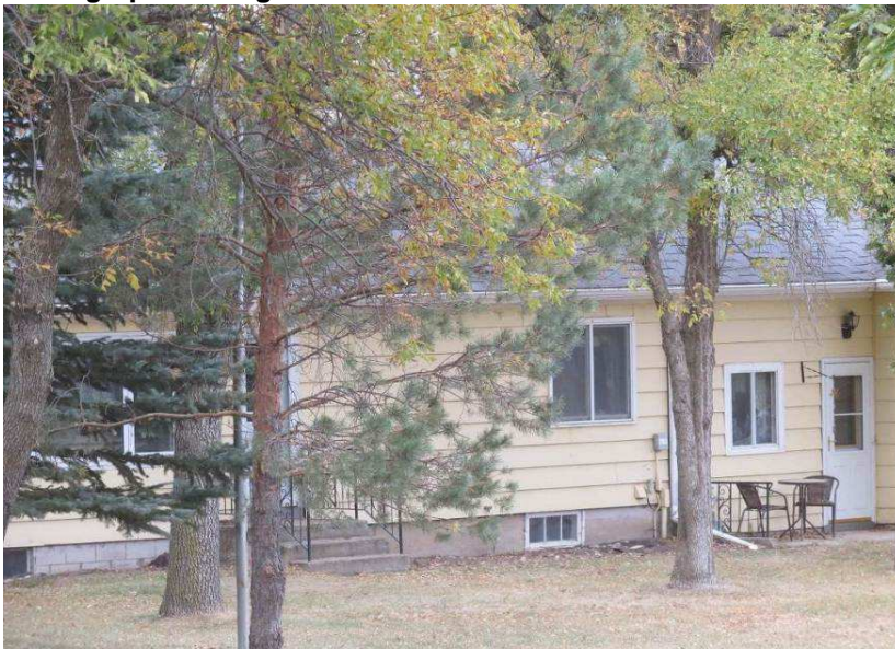
Photograph 4. A view of architectural feature 1 from 158th St NE from west of the farm. Photograph looking NE.
