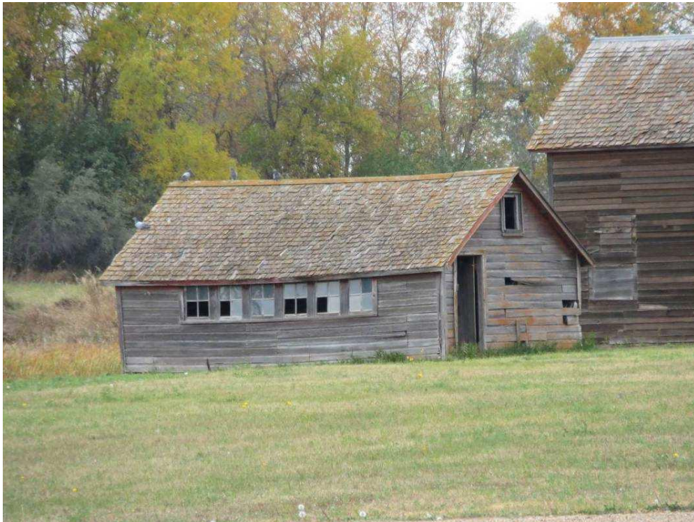
Photograph 10. A view of architectural feature 7 from the south along 279th Ave NE. Photograph looking NW. (Photographer: Adam Holven, Tetra Tech, September 20, 2012.)
