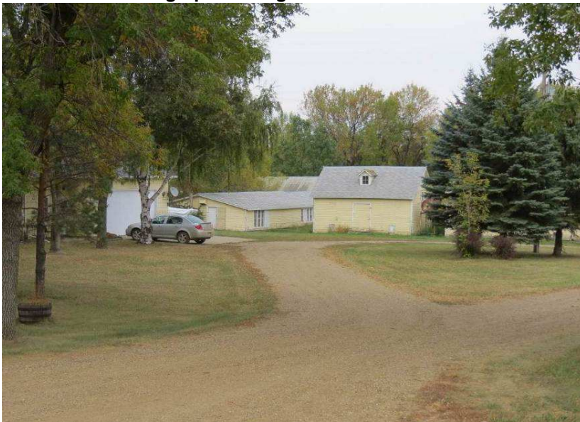
Photograph 6. A view (from left to right) of architectural features 2 and 3 from 158th St NE from west of the farm. Photograph looking NE.
