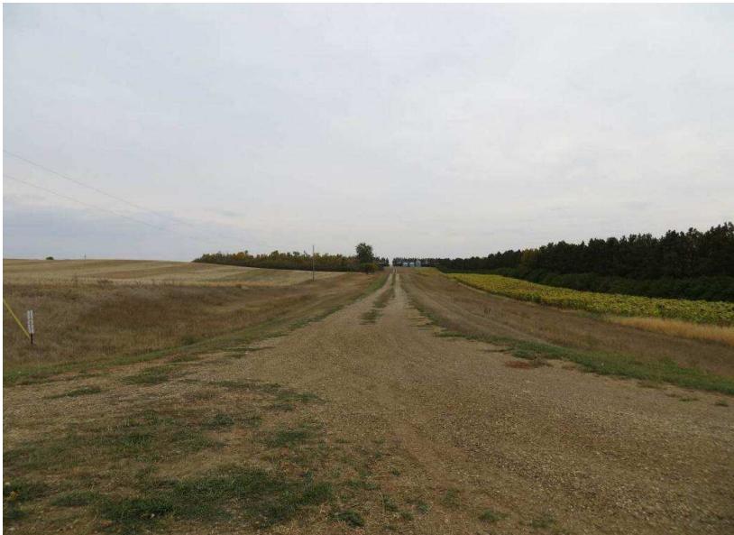
Photograph 2. A view of F6 from 266th Ave NE . Photograph looking S. (Photographer: Adam Holven, Tetra Tech, September 20, 2012.)
