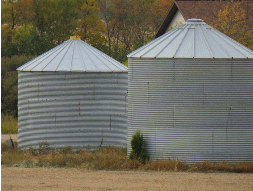
Photograph 13. A view of architectural feature 1 from the southeast along 279th Ave NE. Photograph looking NW.
