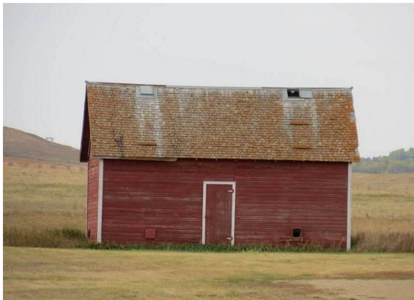
Photograph 22. A view of architectural feature 7 from 240th Ave NE. Photograph looking N.
