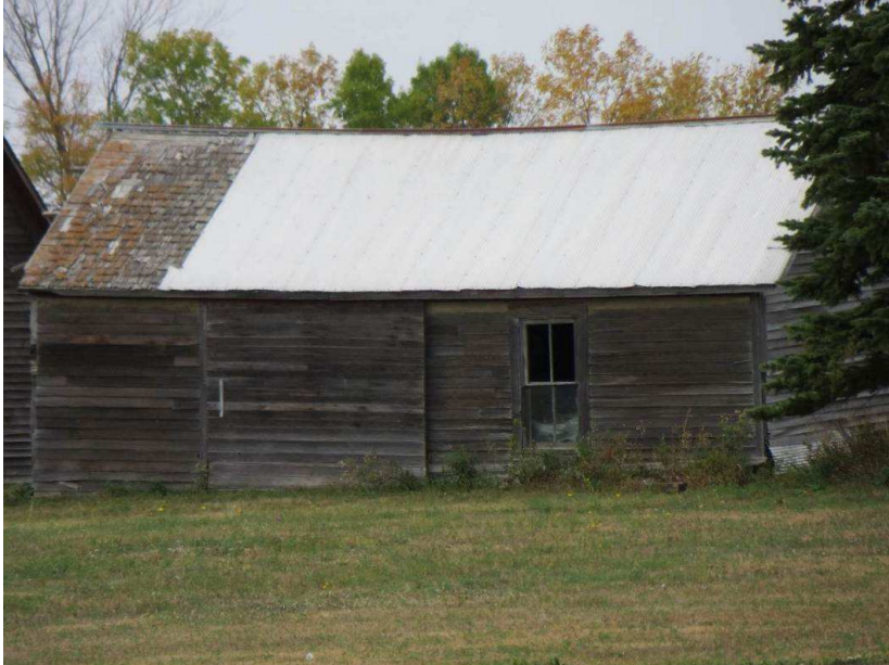
Photograph 8. A view of architectural feature 6 from the south along 279th Ave NE. Photograph looking NW.
