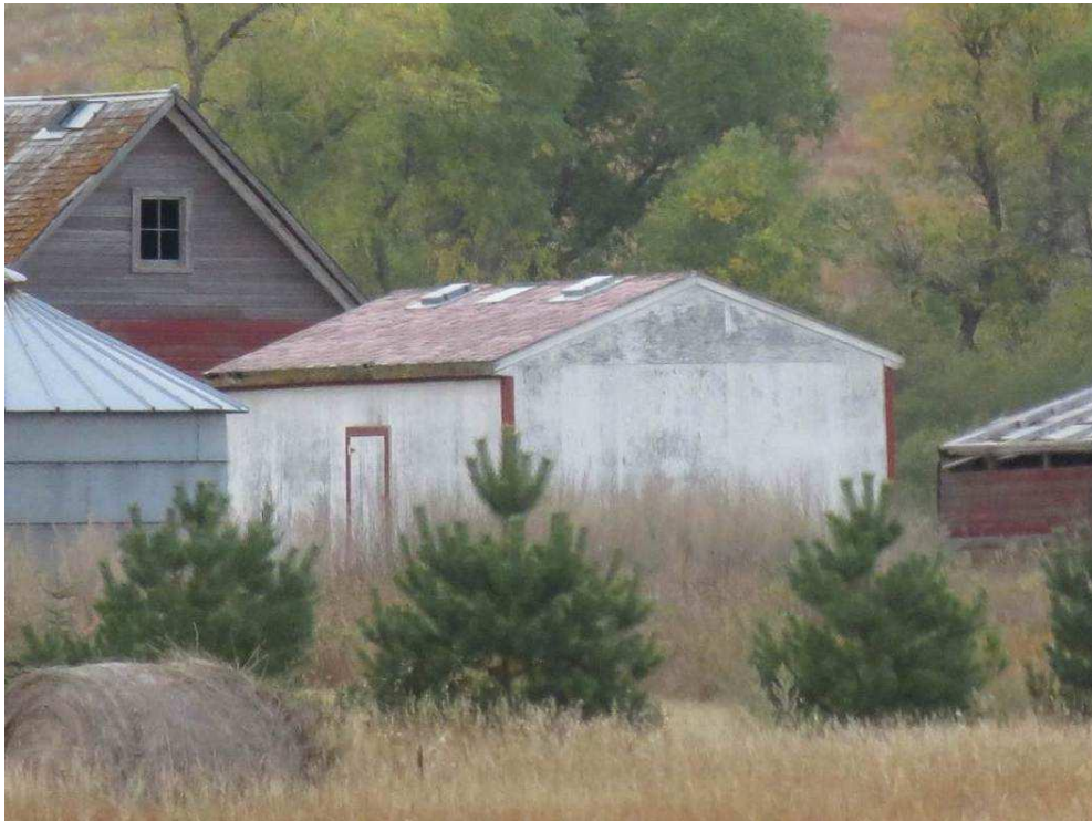
Photograph 50. A view of architectural feature 6 from 240th Ave NE and 171st St NE. Photograph looking NW. (Photographer: Adam Holven, Tetra Tech, September 20, 2012.)
