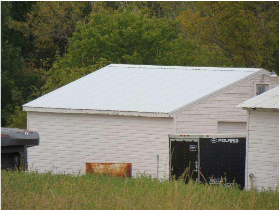
Photograph 96. A view of architectural feature 3 from 158th St NE, southeast of the farm. Photograph looking NW. (Photographer: Adam Holven, Tetra Tech, September 20, 2012.)
