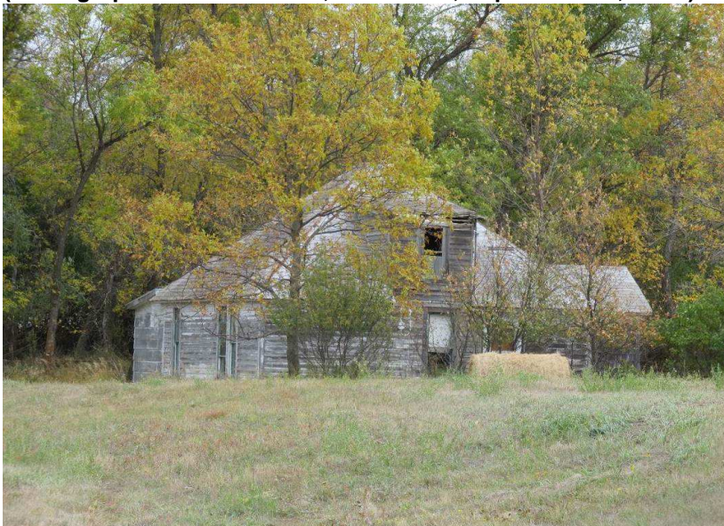
Photograph 4. A view of architectural feature 2 from 171st St NE. Photograph looking SE. (Photographer: Adam Holven, Tetra Tech, September 20, 2012.)
