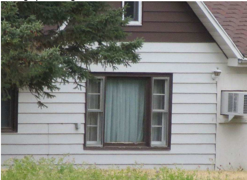
Photograph 6. A view of architectural feature 4 from 158th St NE from east of the farm. Photograph looking NW.
