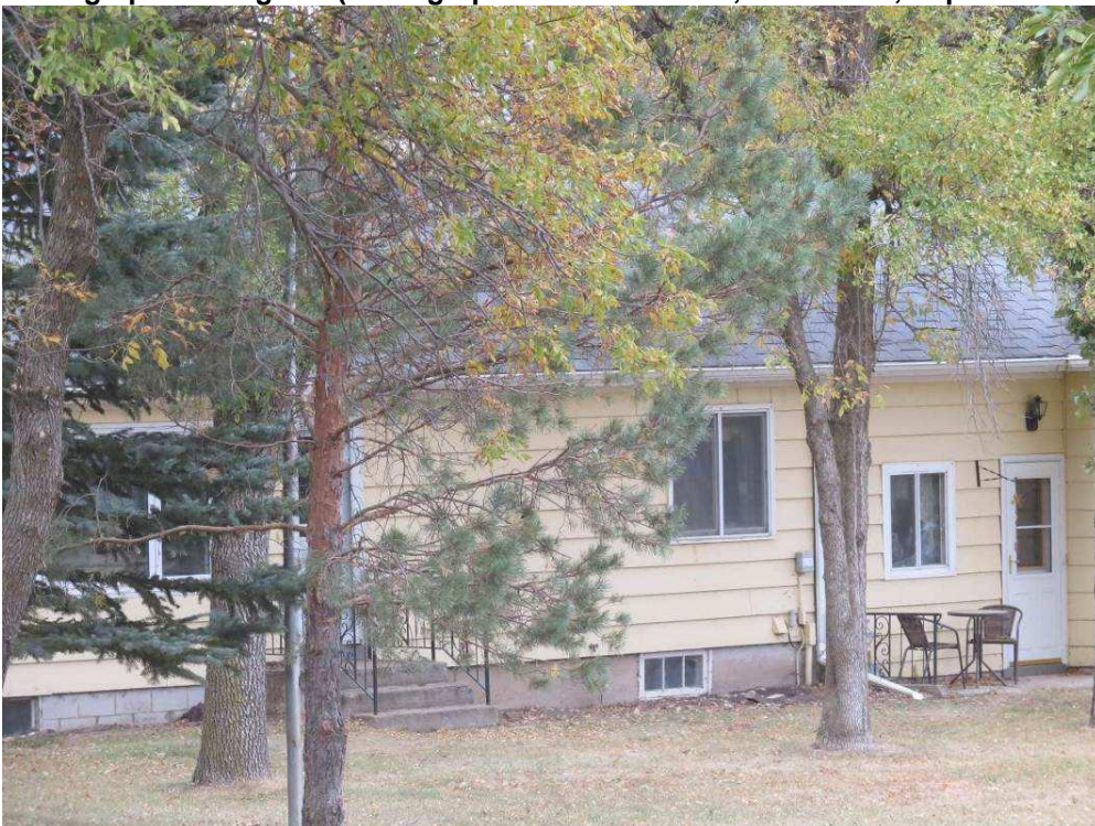
Photograph 80. A view of architectural feature 1 from 158th St NE from west of the farm. Photograph looking NE. (Photographer: Adam Holven, Tetra Tech, September 20, 2012.)
