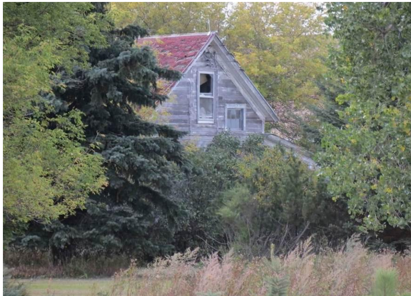
Photograph 9. A view of architectural feature 1 from 240th Ave NE. Photograph looking N-NW.
