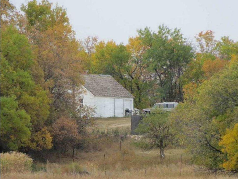
Photograph 106. A view of architectural feature 3 from 266th Ave NE from southwest of the farm. Photograph looking NW. (Photographer: Adam Holven, Tetra Tech, September 20, 2012.)
