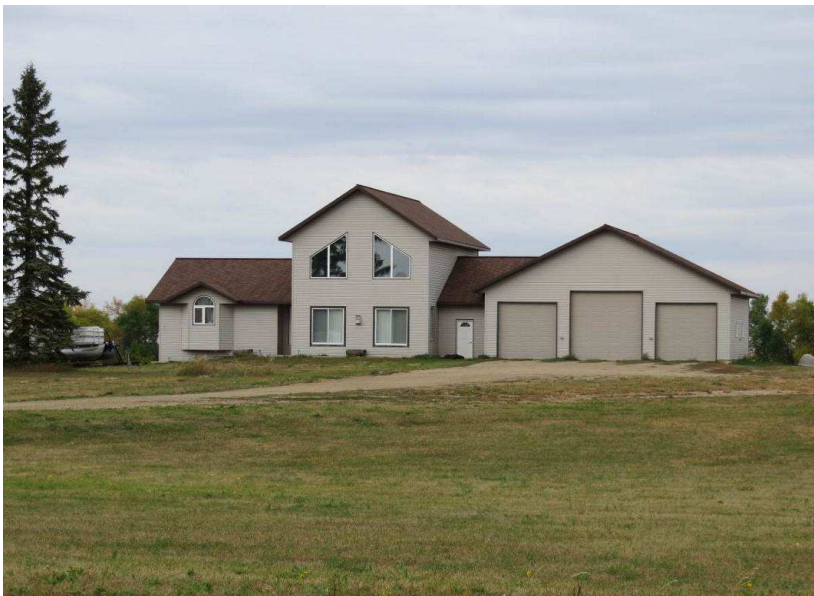
Photograph 4. A view of architectural feature 4 from the south along 279th Ave NE. Photograph looking N.
