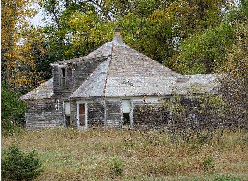
Photograph 3. A view of architectural feature 2 from 266th Ave NE . Photograph looking NE. (Photographer: Adam Holven, Tetra Tech, September 20, 2012.)
