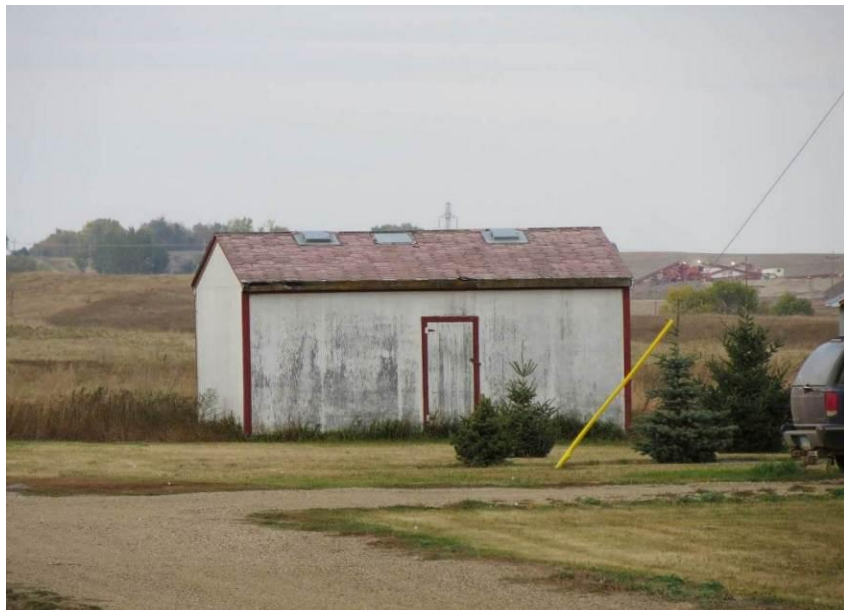
Photograph 23. A view of architectural feature 6 from 240th Ave NE. Photograph looking N-NE.
