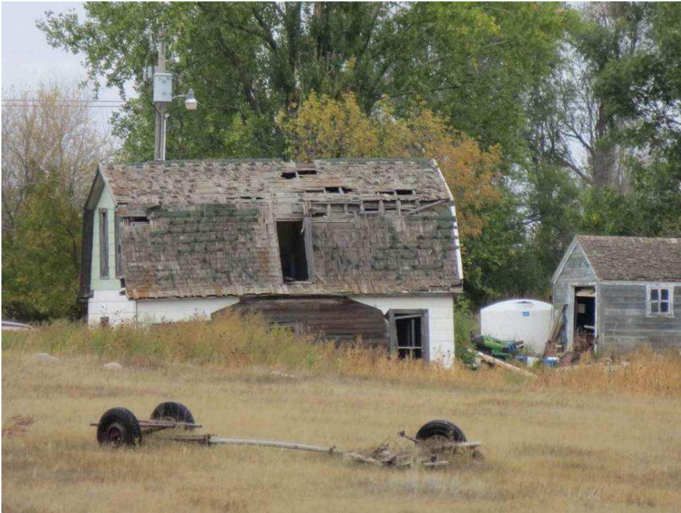
Photograph 69. A view of the former residence from 158th St NE from south of the farm. Photograph looking NNE. (Photographer: Adam Holven, Tetra Tech, September 20, 2012.)
