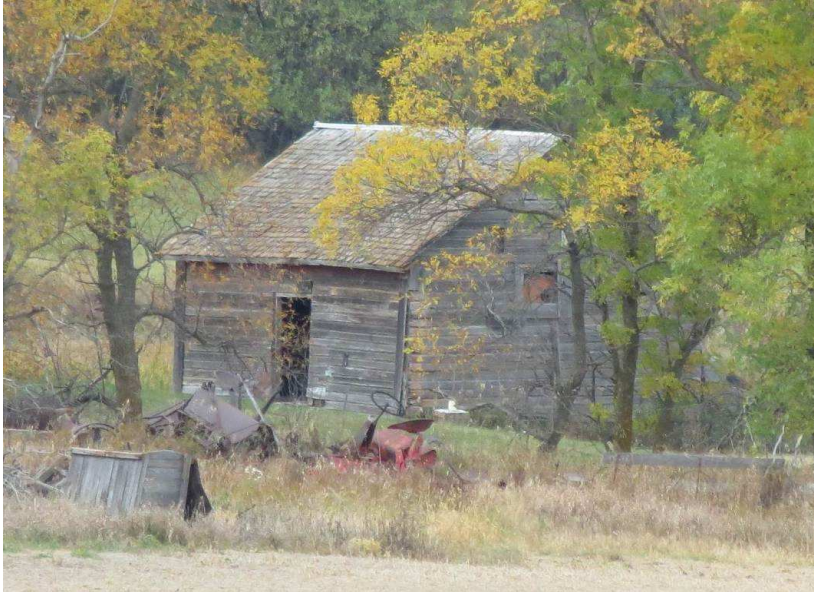
Photograph 5. A view of architectural feature 2 from the southeast along 279th Ave NE. Photograph looking NW.
