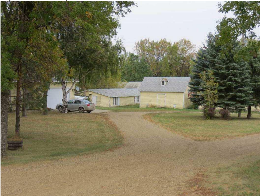
Photograph 82. A view (from left to right) of architectural features 2 and 3 from 158th St NE from west of the farm. Photograph looking NE. (Photographer: Adam Holven, Tetra Tech, September 20, 2012.)
