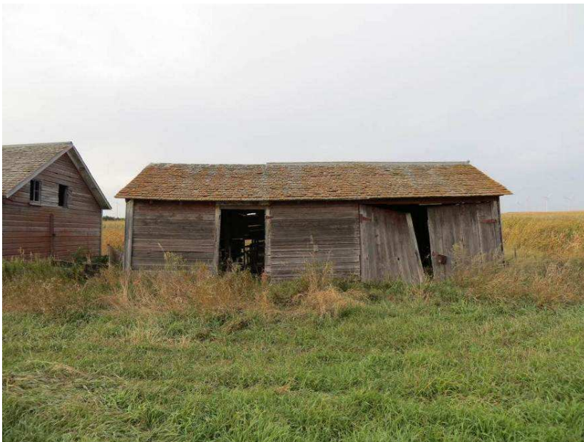
Photograph 8. A view of architectural feature 3 from 240th Ave NE south of the site. Photograph looking N.
