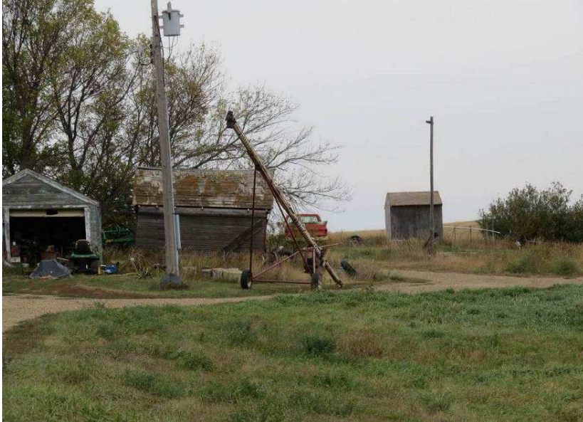
Photograph 17. A view (from left to right) of architectural features 9, 8, and 10 from 158th St NE from west of the farm. Photograph looking E.
