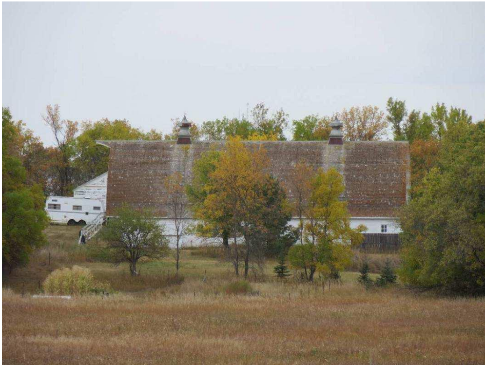
Photograph 108. A view of architectural feature 4 from 266th Ave NE, south of the farm. Photograph looking N-NW. (Photographer: Adam Holven, Tetra Tech, September 20, 2012.)
