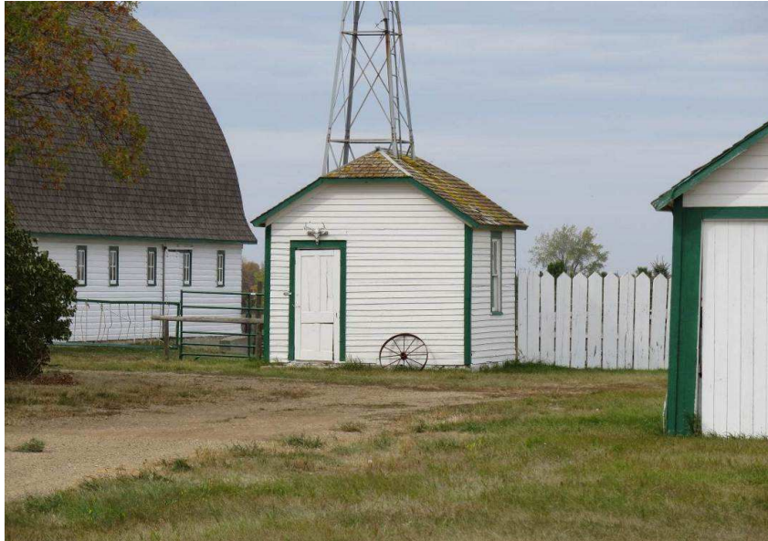
Photograph 7. A view of architectural feature 6 (flanked by features 3 and 5) from 266th Ave NE. Photograph looking NNW. (Photographer: Adam Holven, Tetra Tech, September 20, 2012.)
