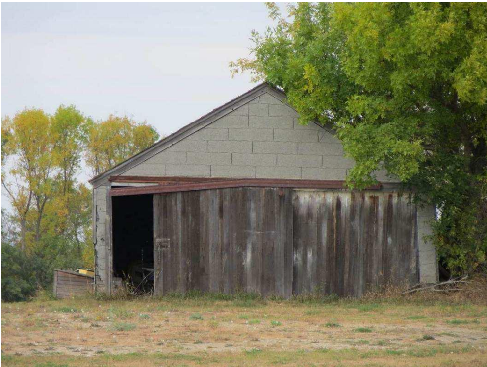
Photograph 7. A view of architectural feature 3 from the south along 279th Ave NE. Photograph looking N. (Photographer: Adam Holven, Tetra Tech, September 20, 2012.)
