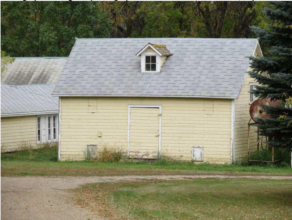
Photograph 84. A view of architectural feature 3 from 158th St NE from west of the farm. Photograph looking NE. (Photographer: Adam Holven, Tetra Tech, September 20, 2012.)
