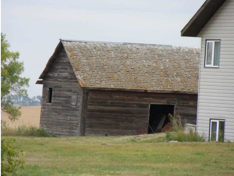
Photograph 7. A view of architectural feature 5 and the corner of architectural feature 4 (at right) from the southwest along 279th Ave NE. Photograph looking NE.
