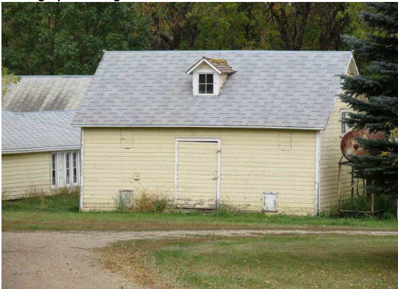
Photograph 8. A view of architectural feature 3 from 158th St NE from west of the farm. Photograph looking NE.
