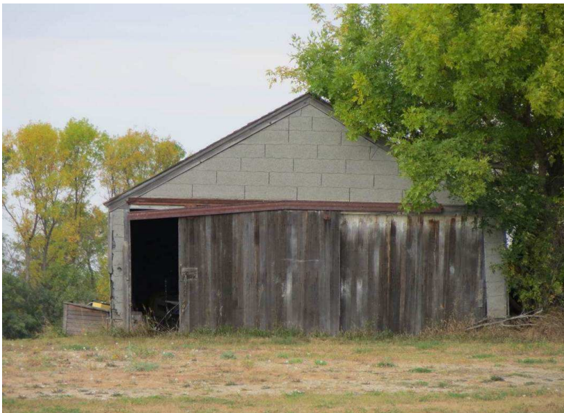
Photograph 6. A view of architectural feature 3 from the south along 279th Ave NE. Photograph looking N.
