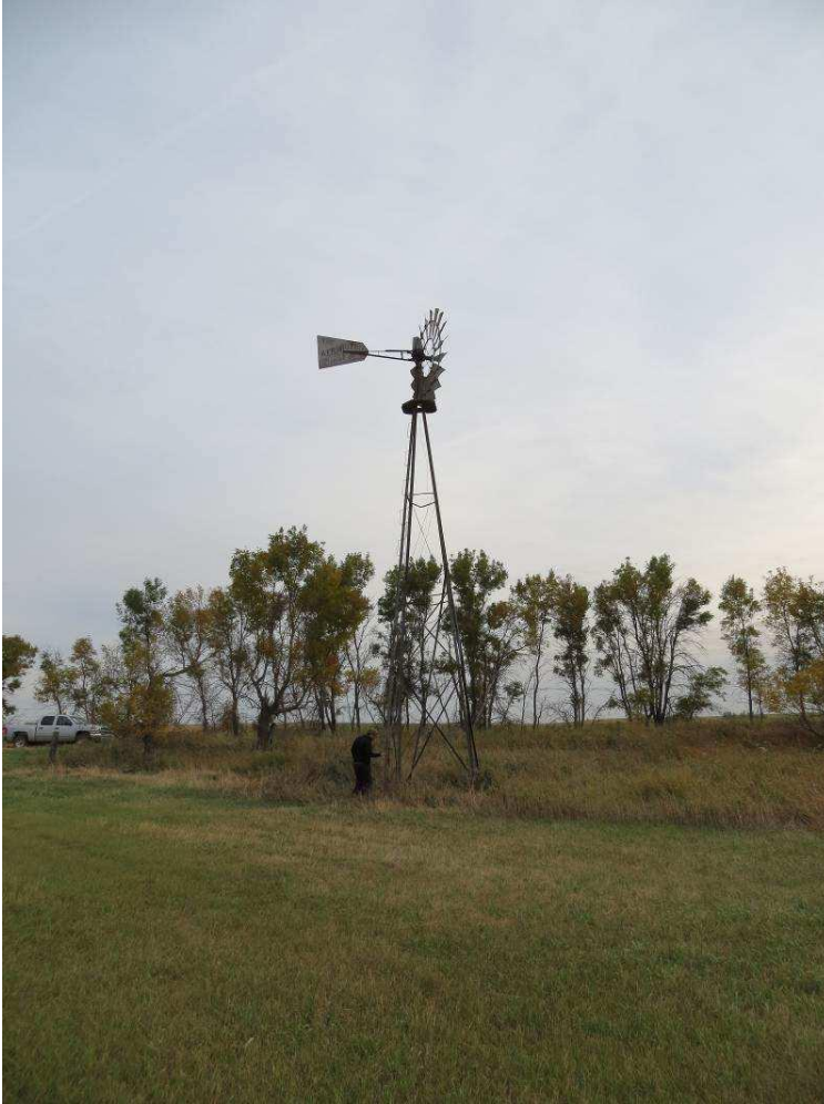
Photograph 121. A view of architectural feature 7. Photograph looking NW. (Photographer: Adam Holven, Tetra Tech, September 20, 2012.)
