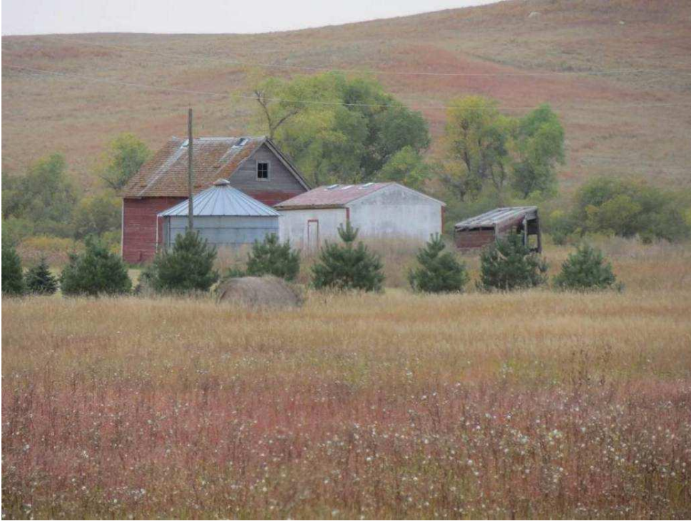
Photograph 48. A view of architectural features 7, 5, 6, and 15 (left to right) from 240th Ave NE and 171st St NE. Photograph looking NW. (Photographer: Adam Holven, Tetra Tech, September 20, 2012.)
