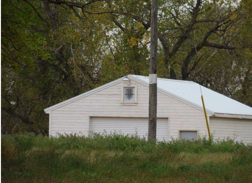
Photograph 11. A view of architectural feature 3 from 158th ST NE, northeast of the farm. Photograph looking SW.
