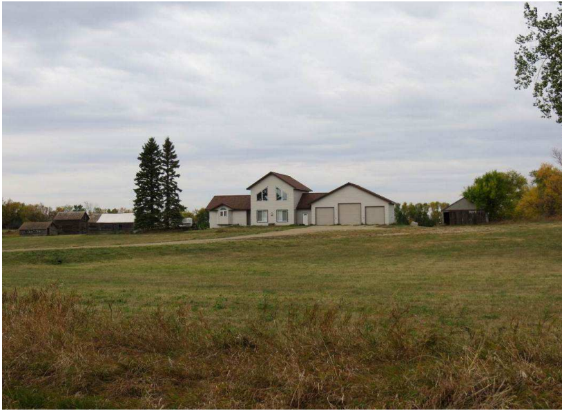
Photograph 3. A view of F1 from the south along 279th Ave NE. Photograph looking N.
