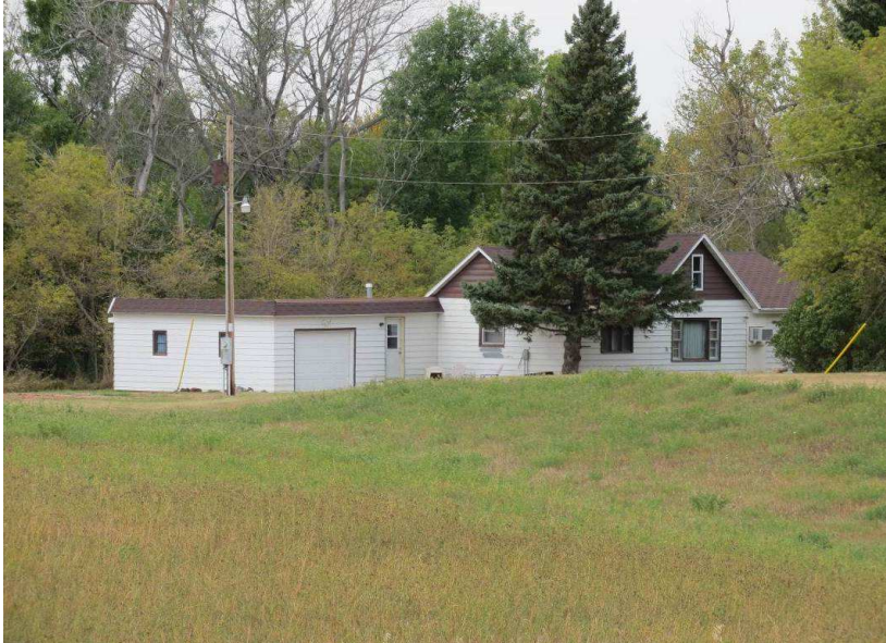
Photograph 5. A view of architectural feature 4 from 158th ST NE from east of the farm. Photograph looking NW.
