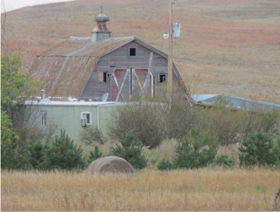
Photograph 40. A view of architectural features 2 (barn) and 9 (mobile home) from 240th Ave NE. Photograph looking NW. (Photographer: Adam Holven, Tetra Tech, September 20, 2012.)
