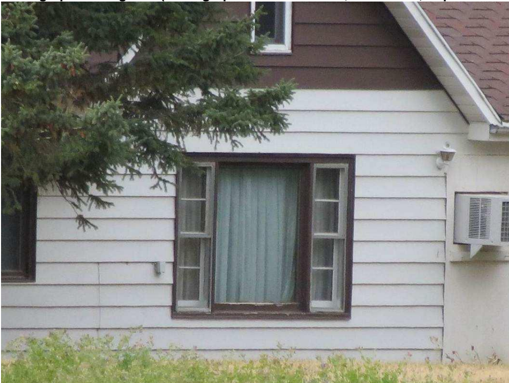
Photograph 92. A view of architectural feature 4 from 158th St NE from east of the farm. Photograph looking NW. (Photographer: Adam Holven, Tetra Tech, September 20, 2012.)
