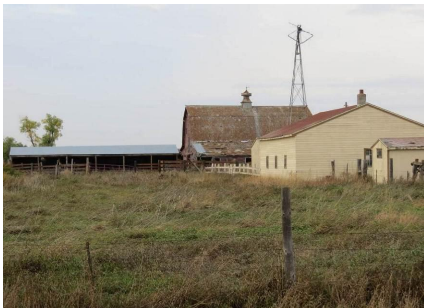
Photograph 6. A view of the west side of F5 from 240th Ave NE. Photograph looking N.
