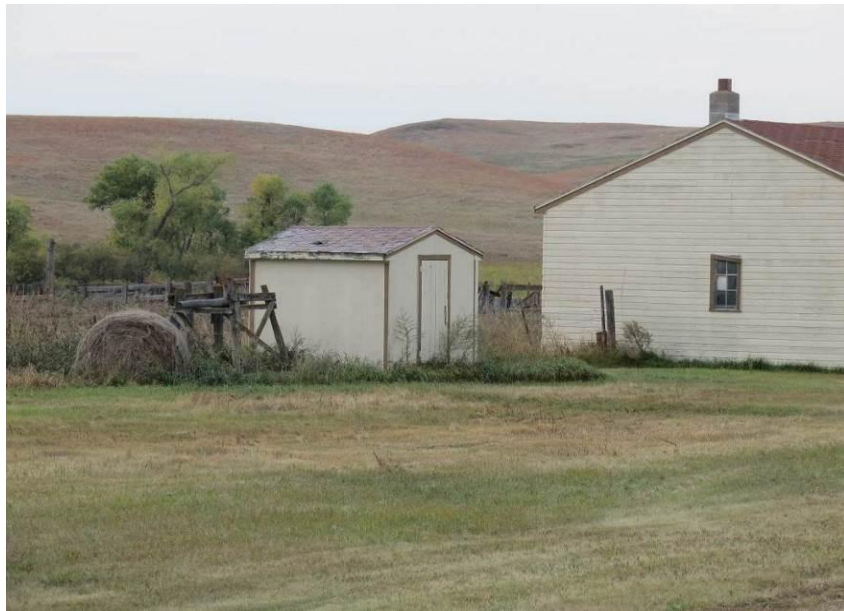
Photograph 15. A view of architectural feature 14 (left) and 11 from 240th Ave NE. Photograph looking NW.
