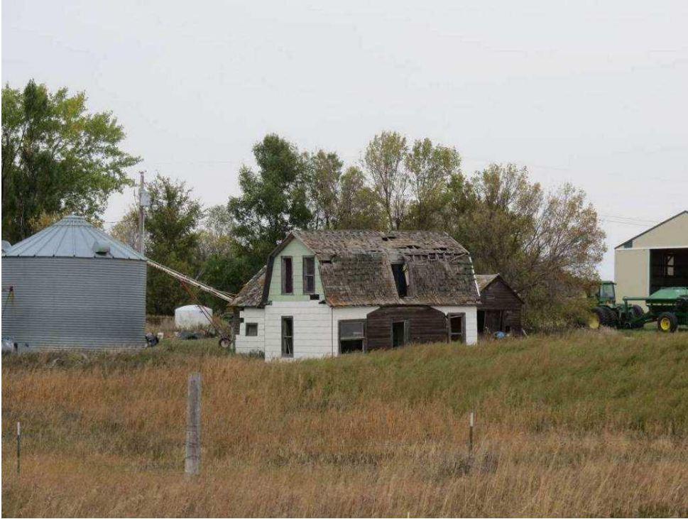
Photograph 68. A view (from left to right) of architectural features 6, 5, 8, and 2 from 158th St NE from south of the farm. Photograph looking NE. (Photographer: Adam Holven, Tetra Tech, September 20, 2012.)
