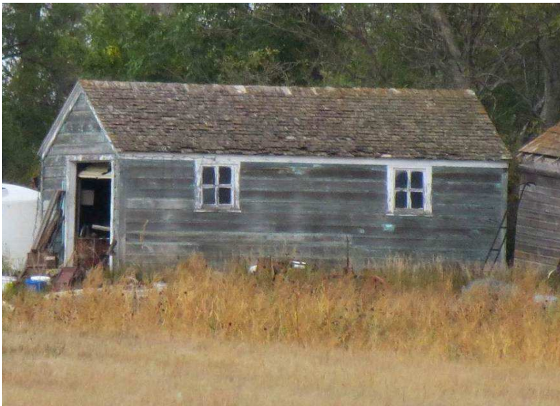
Photograph 16. A view of architectural feature 9 from 158th St NE from south of the farm. Photograph looking NNE.
