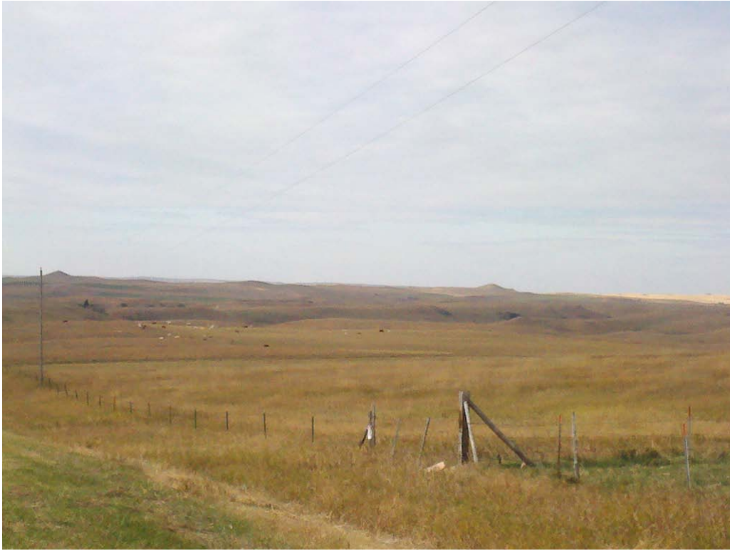
Photo 1. General topography within the Allele Wind Resource Area.
