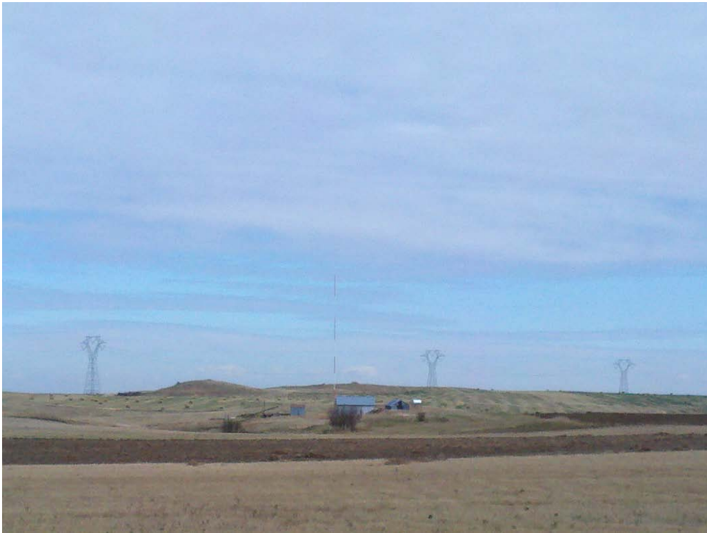
Photo 9. Meteorological tower and powerline located within the Allele Wind Resource Area.
