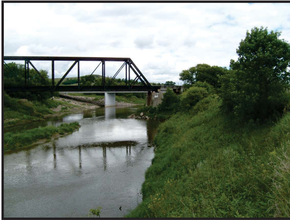
Photo 53: Heart River (Site 24) a WOUS, facing north (6/20/2012).
