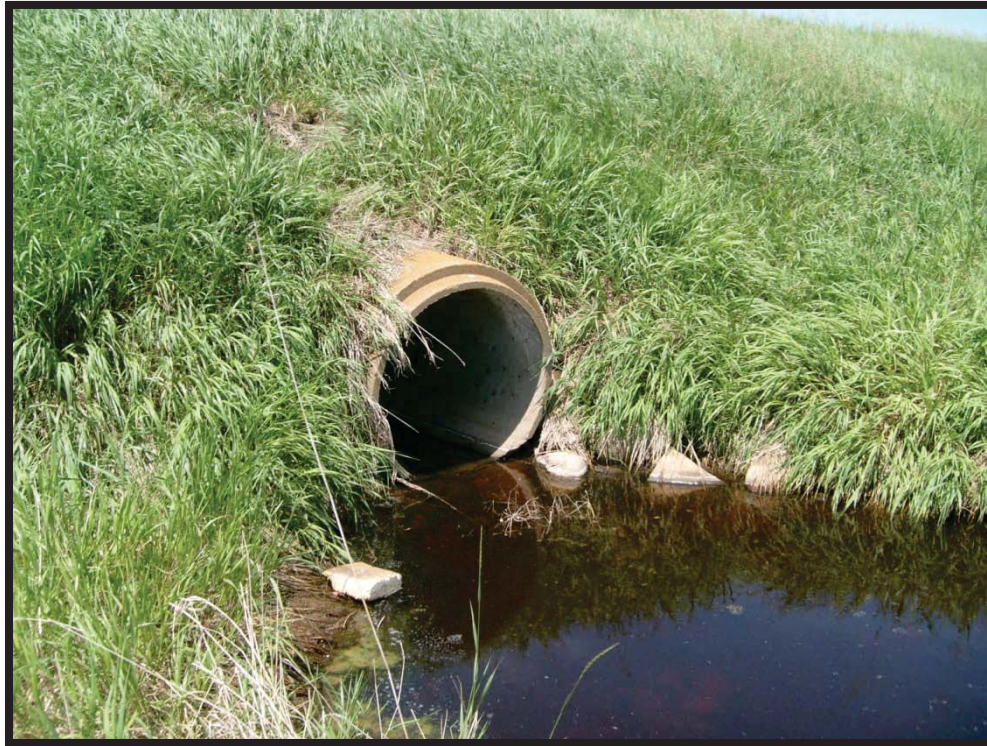
Photo 39: Site 16, facing northwest, culvert (6/22/2012).
