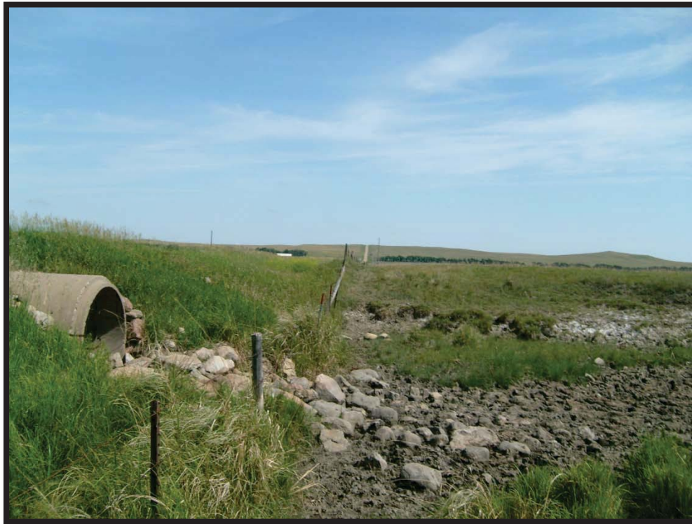
Photo 51: Site 22 (an oxbow of the Little Heart River), facing north (6/23/2012).
