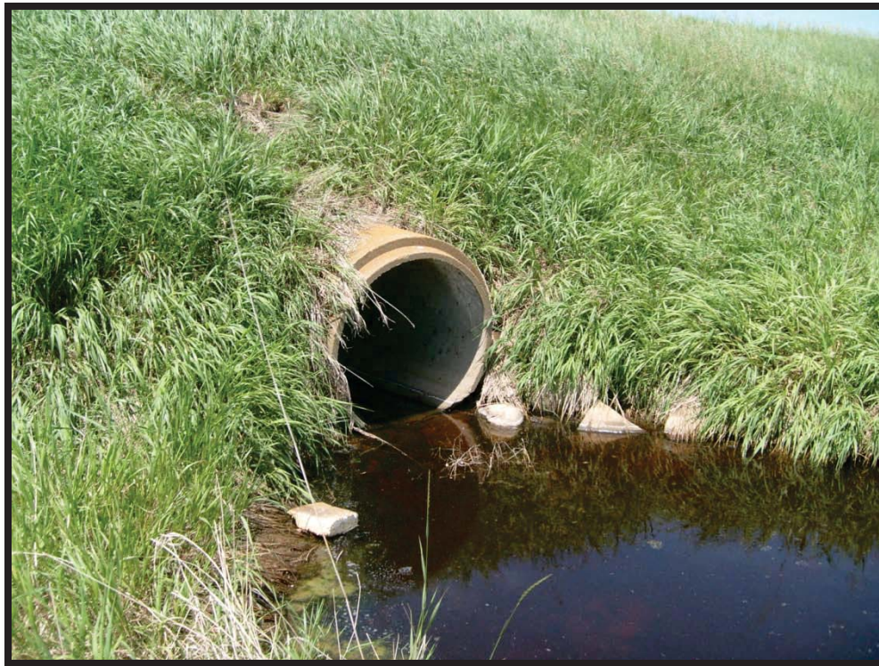
Photo 39: Site 16, facing northwest, culvert (6/22/2012).
