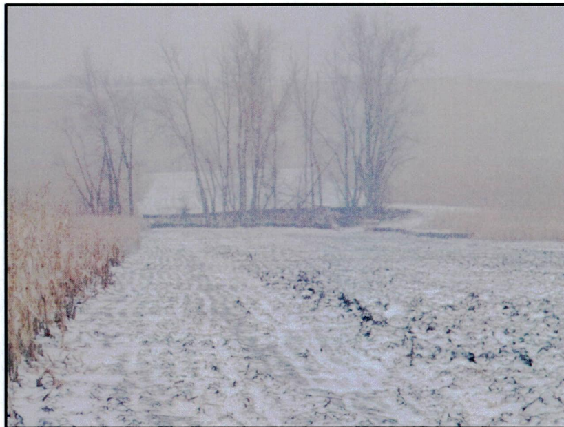
Photo 6. Direction: North (GPS Point #62). Pipeline bored underneath non-jurisdictional wetland with minimal impact.
