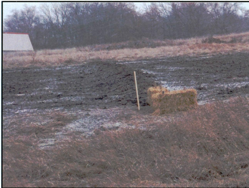
Photo 8. Direction: West (GPS Point #8). Slope breaker.
