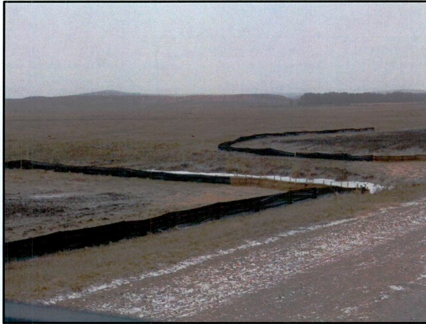
Photo 7. Direction: Northwest (GPS Point #6). Pipeline bored underneath the Little Heart River.
