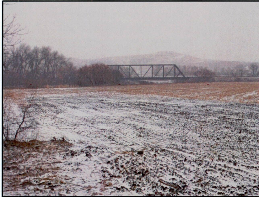
Photo 9. Direction: North (GPS Point #52). South end of bore passing under the Heart River, BNSF Railroad, and I-94 Business Loop.
