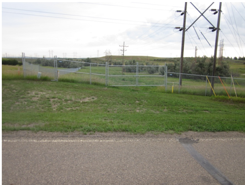
Below: Image 6, Pipeline Crossing into Heskett Station Property
