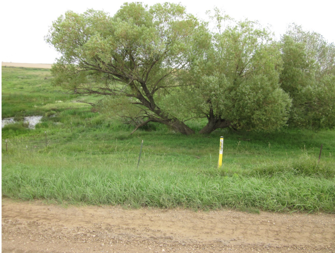
Below: Image 12, Wetland Crossing, Bore Pipe No. 15
