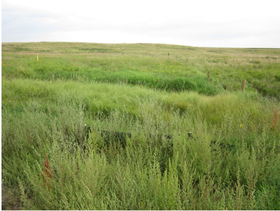
Above: Image 9, Wetland Crossing Bore Pipe No. 8 close to stream
