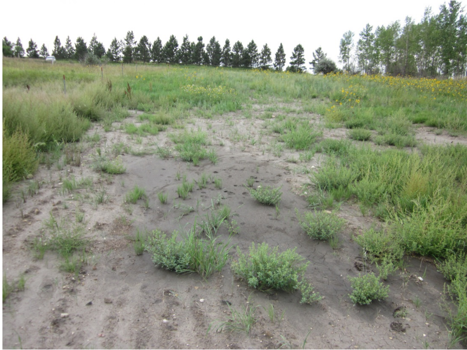
Above: Image 19, Area of Concern (same as above)- Wetland Crossing Bore Pipe No.8
