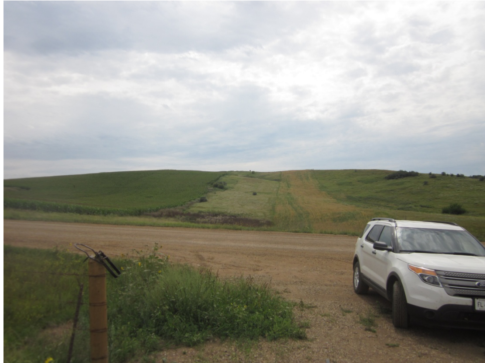
Above: Image 25, ROW crosses Cty Rd 82, Bore Pipe No. 15 to block valve
