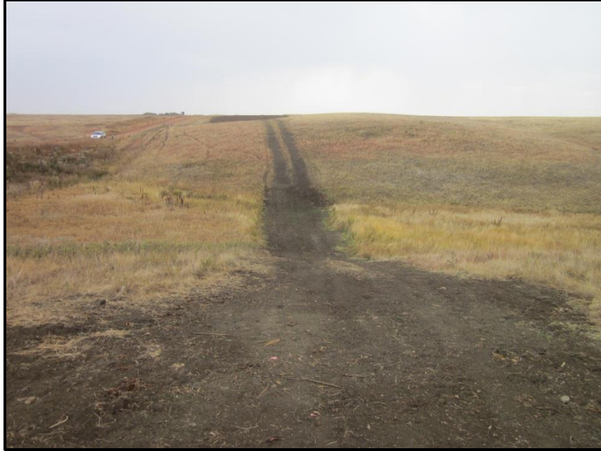
Photo 13. Direction: West. Just south of 49 th St., view of the pipeline where it was bored under a wetland. No sedimentation to the wetland was noted, but vegetation had been disturbed by vehicle traffic.
