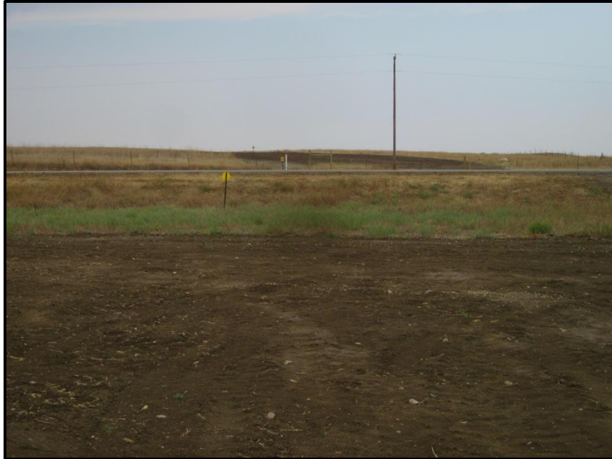
Photo 5. Direction: West. View shows the road bore of County Highway 5 on the east side. No settling to the roadway was noted. Note the three posted signs: on the east and west side of the roadway, and one near the fenceline on the west side.
