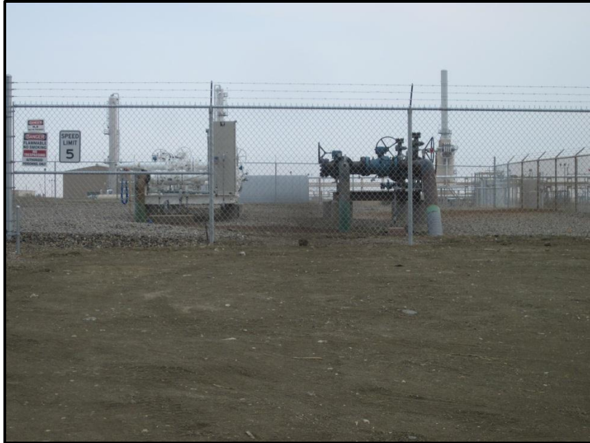
Photo 1. Direction: North. View of the beginning of the pipeline at the Stateline Gas Plant in Williams County, North Dakota. Note posted warning signage and fence surrounding block valve, which is located at the launcher barrel.
