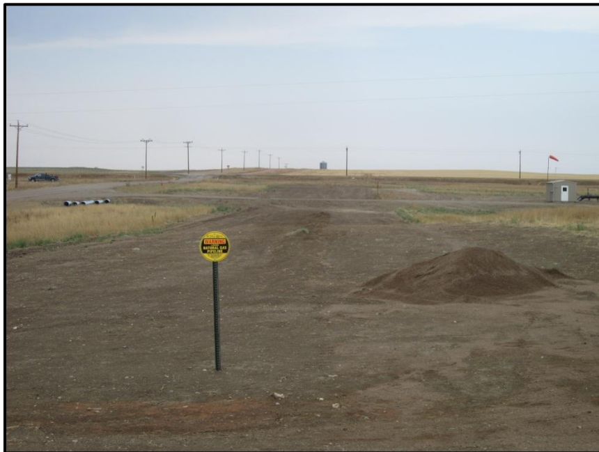
Photo 2. Direction: West. View of the pipeline as it leaves the processing plant. The driveway to the plant was bored. Note the posted warning signage.
