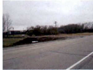
Access at ND 20 and 52nd Increased Radius for Transport Delivery of Tower, Blades, and Nacelle
