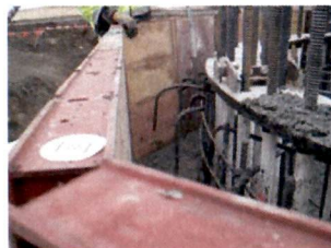
Pier Formwork and Tower Base Ring 14' Diameter
