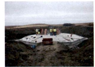
Forming the Turbine Pier Assembly on the Concrete Foundation 48' in Width
