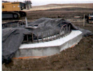
Concrete Pier Backfilled
