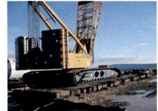
Assembly Crane Erected and Supported with Cribs
