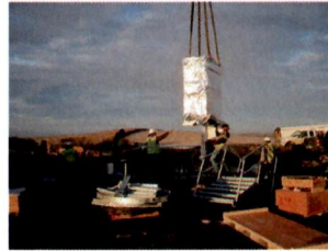
DTU (Down Tower Unit) Electrical Component Set on Platform and Pier
