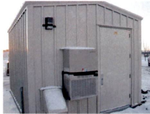
Control Hut Delivered and Set for Switchgear and Interconnect
