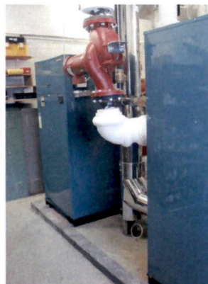
New Boilers (3) Complete, Insulated Domestic Hot Water Tanks Complete
