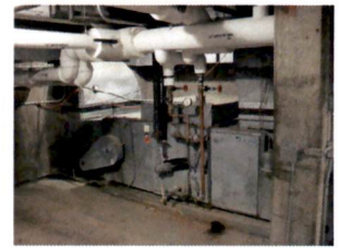
Insulated and Labeled Mechanical Systems Complete
