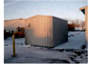
Control Hut In Line with Electrical Collector Assembly
