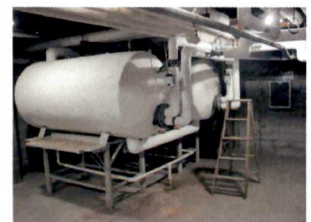
New Boilers (3) Complete, Insulated Domestic Hot Water Tanks Complete
