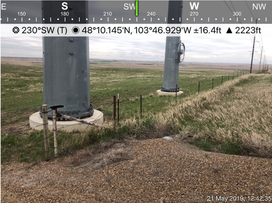
Photo 6 – Base of Structures in Segment A
