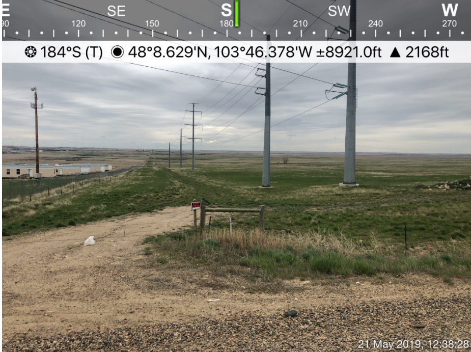
Photo 5 – Segment A Structures in Pastureland
