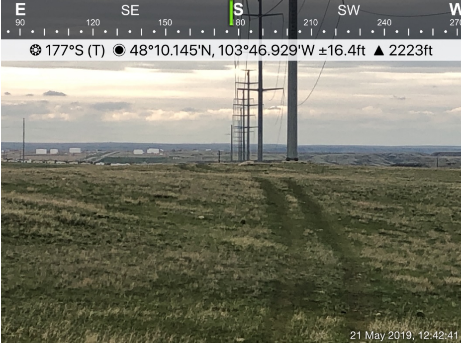
Photo 7 – Segment A Right-of-Way
