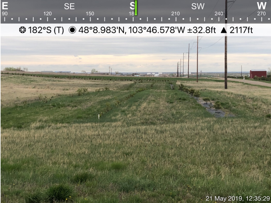
Photo 3 – Tree Planting Surrounding Outside of Judson Substation
