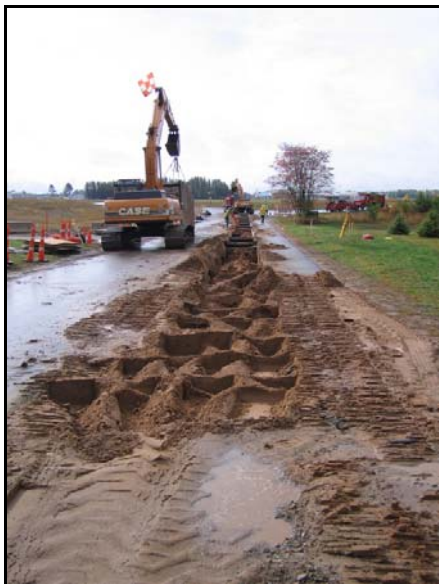
Figure 16 Backfilling and Street Restoration
