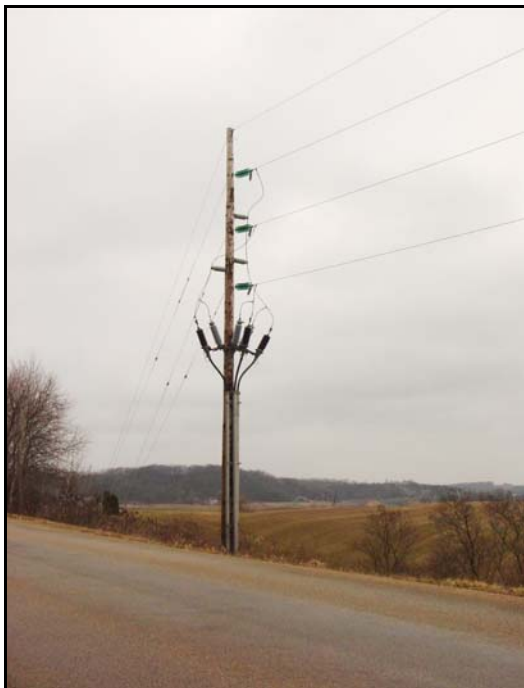
Figure 5 138 kV Underground to Overhead Transition Structures
