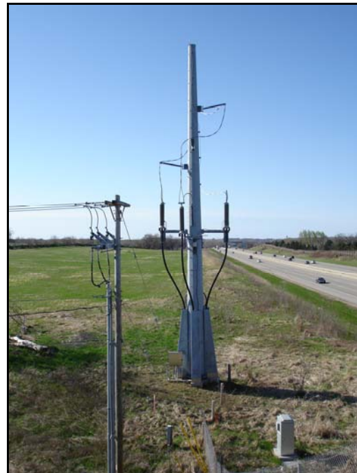
Figure 5 138 kV Underground to Overhead Transition Structures
