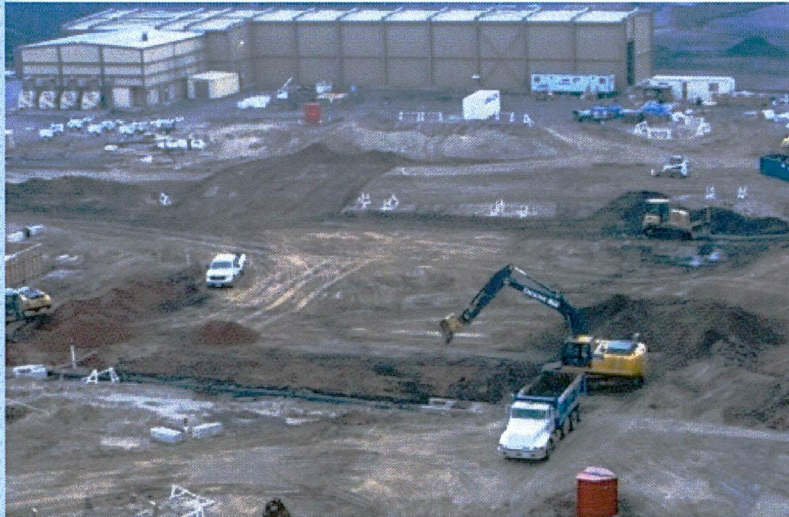
5-29 Baghouse and CFB excavation
