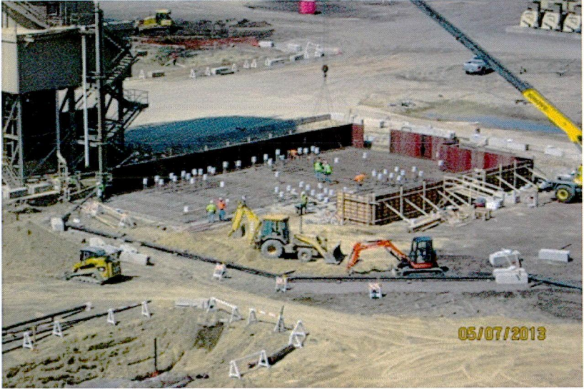
5-07 Foundation rebar placement
