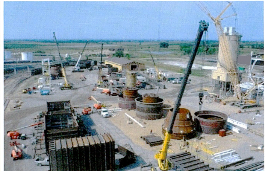
8-21 Plant south view
