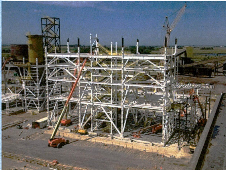
8-29 CFB & start of baghouse steel erection
