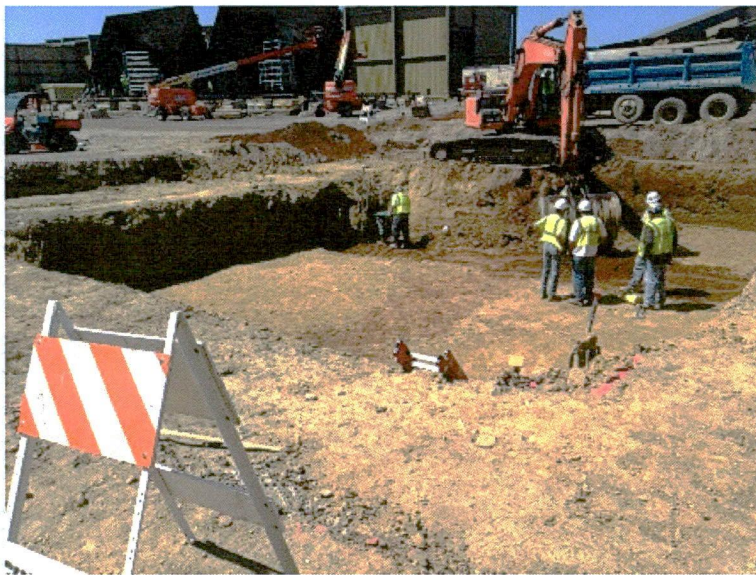
8-09 Excavating ID fan area
