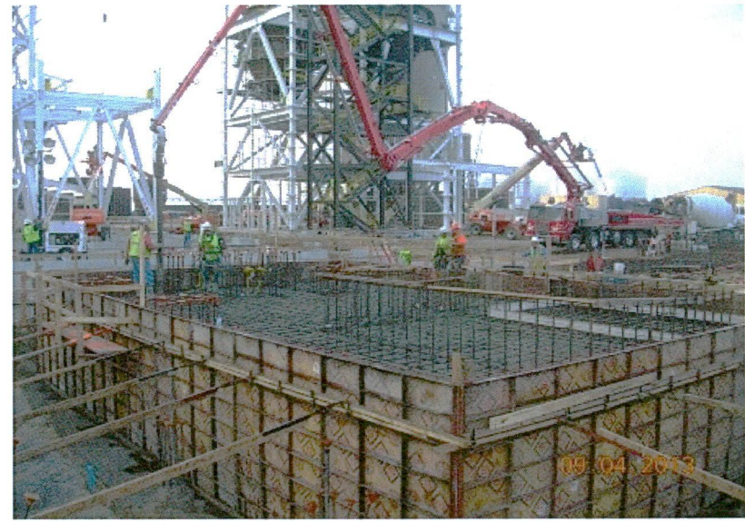
ID Fan B foundation placing concrete
