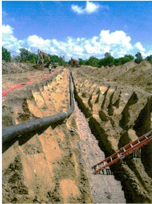
8-05 Low quality water pipeline
