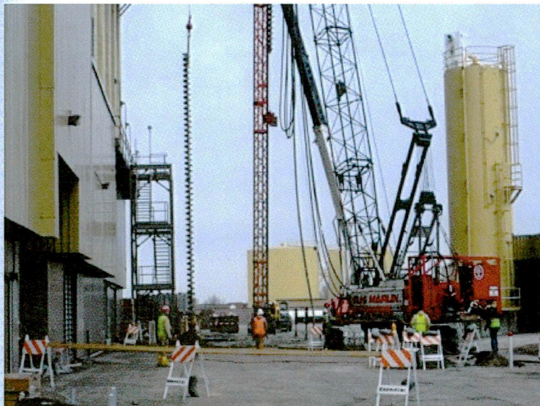
5-01 North production piles
