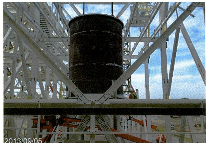
9-05 Waste ash bin lowered
