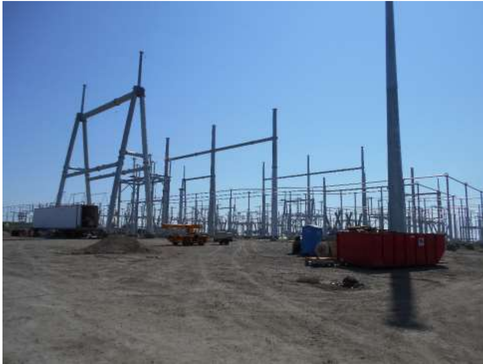
Photo 1 –Overall site picture looking southeast.
