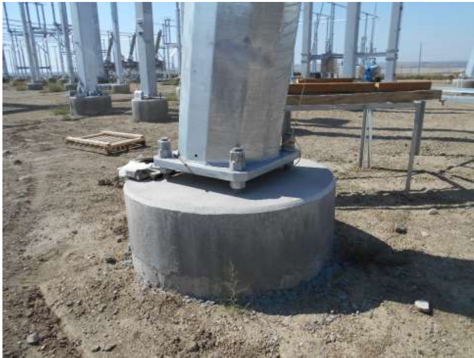
Picture 3 – Typical structural pier and mounting bolts.
