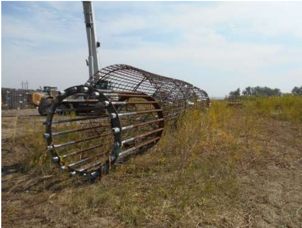
Photo 5 – Steel Rebar for concrete structure base.
