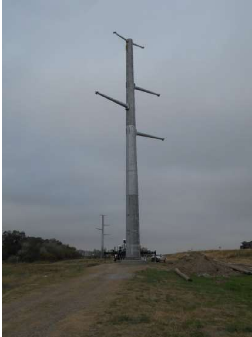
Photo 1 -Typical Galvanized Type of Structure.
