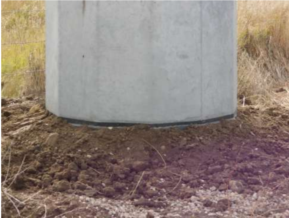
Photo 3 - Typical Embedded Type Structural Base.
