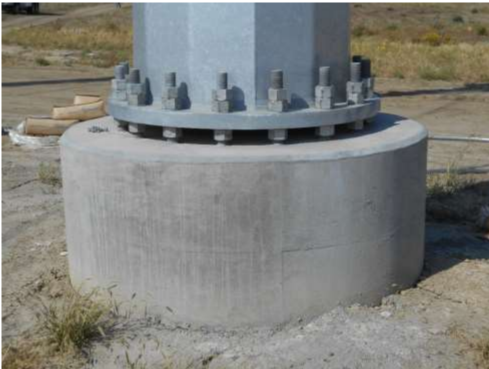
Photo 4 - Typical Concrete Type Structural Base.
