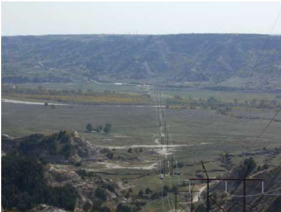
Photo 6 – Transmission line crossing Little Missouri River (looking south).
