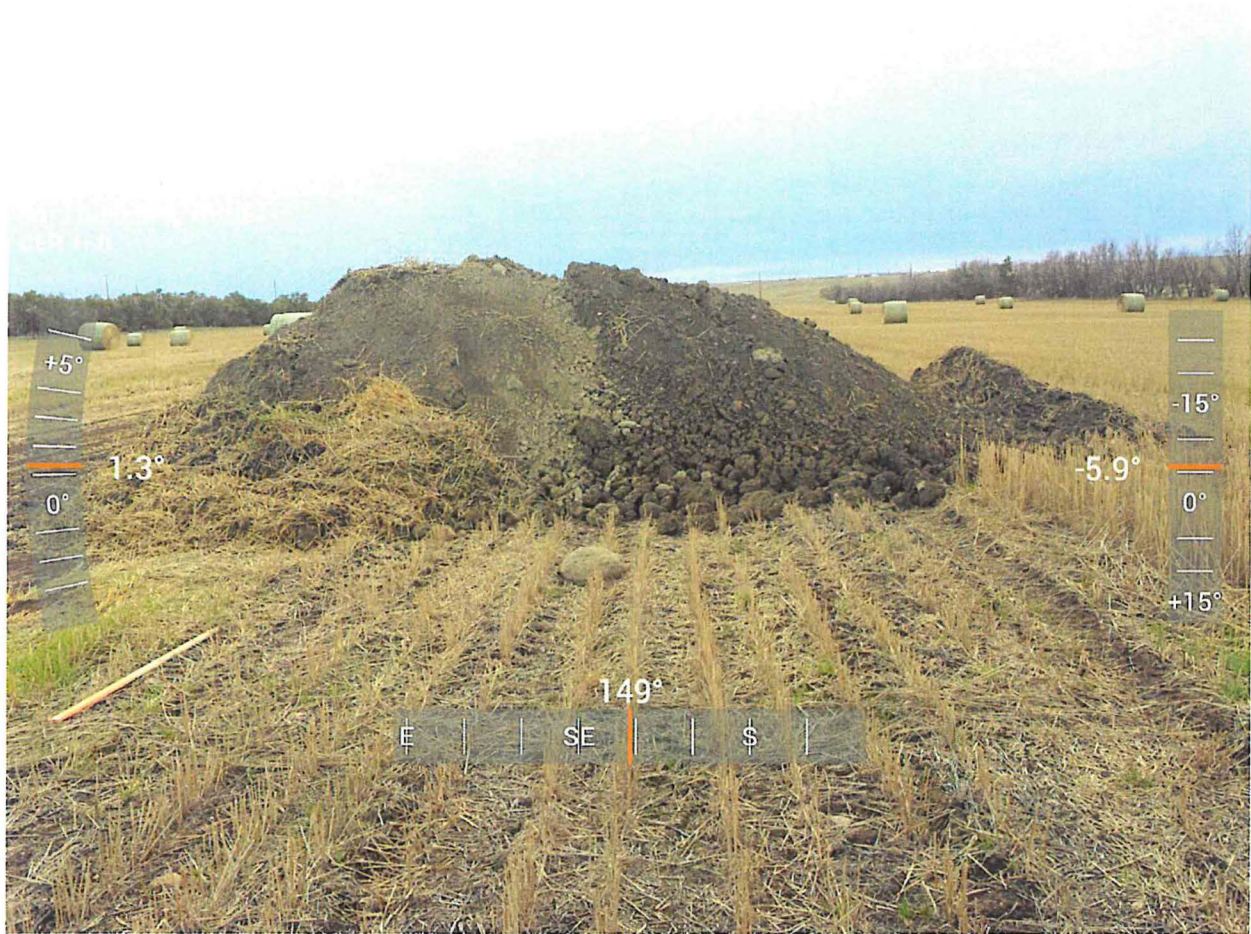
Photo 5 – Soil pile from foundation construction to be used for fill.
