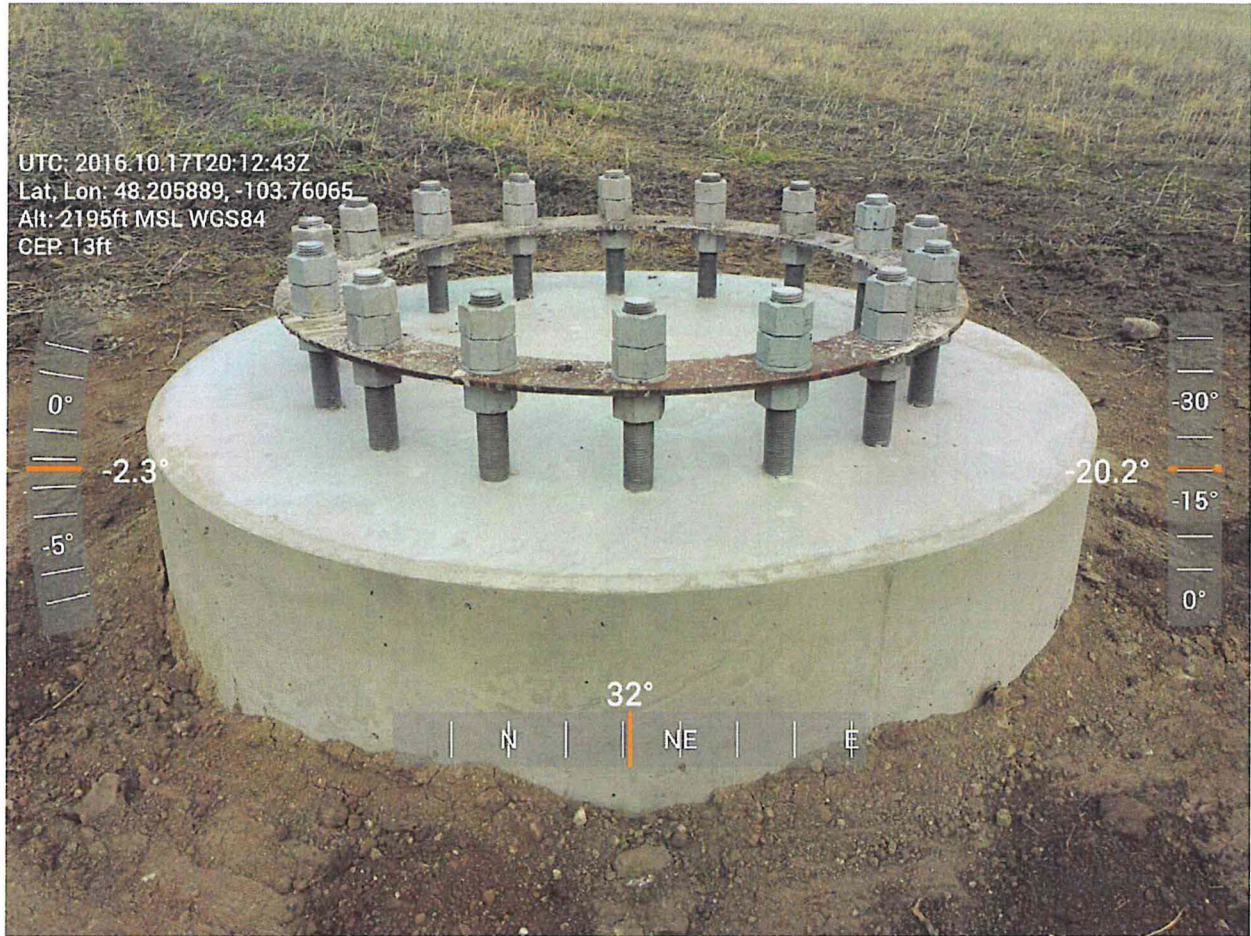
Photo 3 -Typical concrete type structural base.
