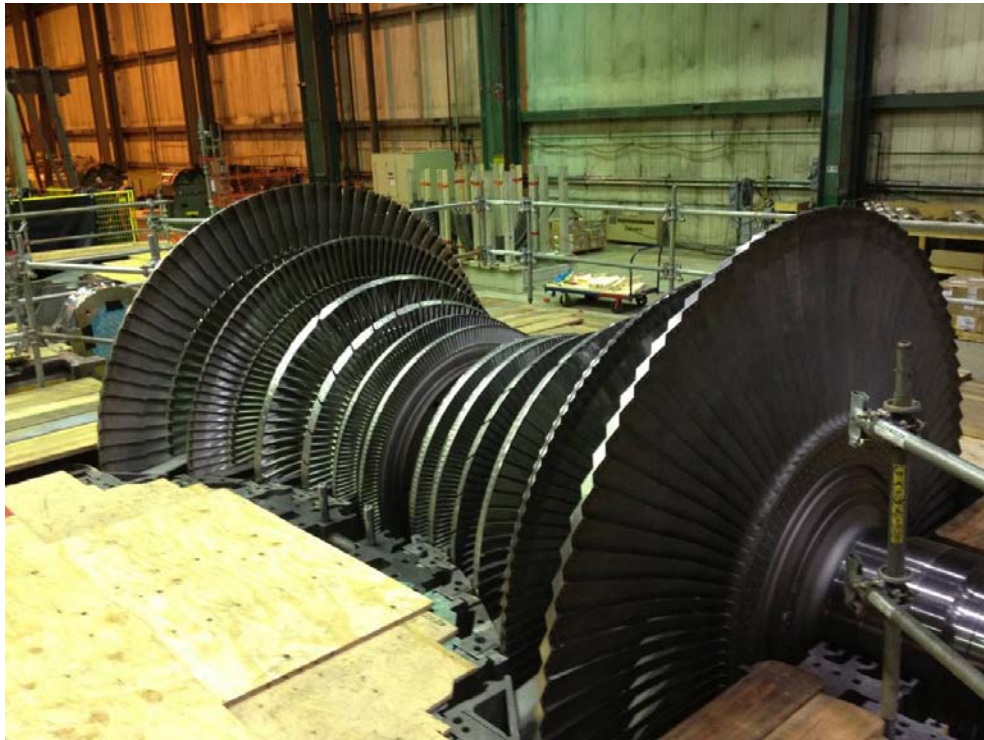
LP-A rotor successfully installed on May 1, 2013.
